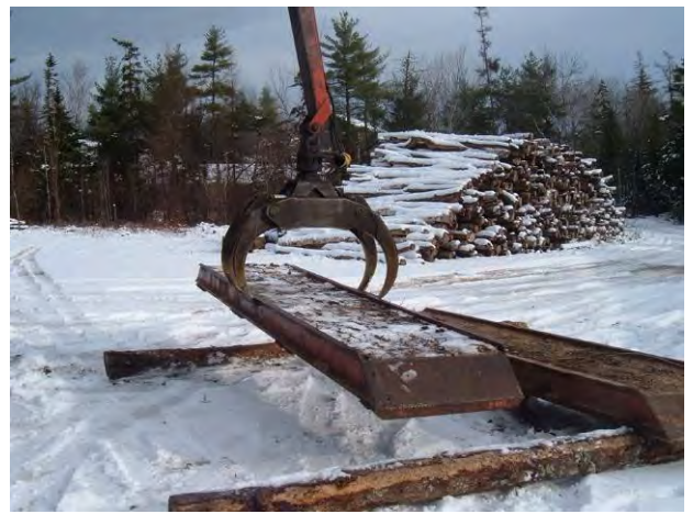
Practice set-up of a temporary watercourse crossing using bunk logs and fabricated runners.
