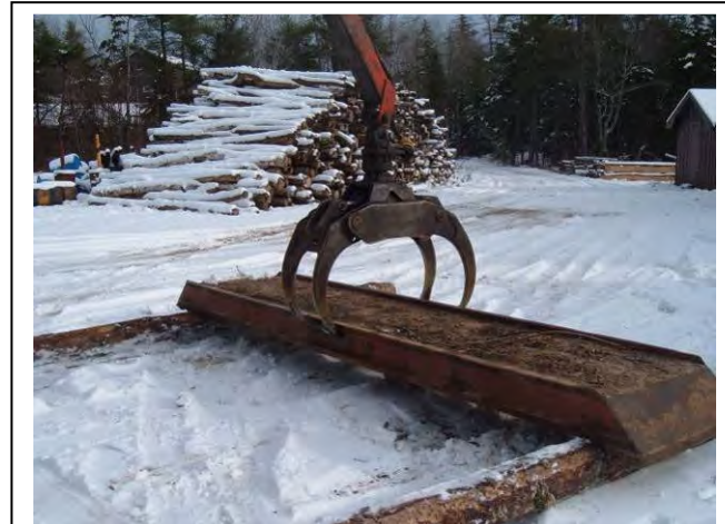
Practice set-up of a temporary watercourse crossing using bunk logs and fabricated runners.
