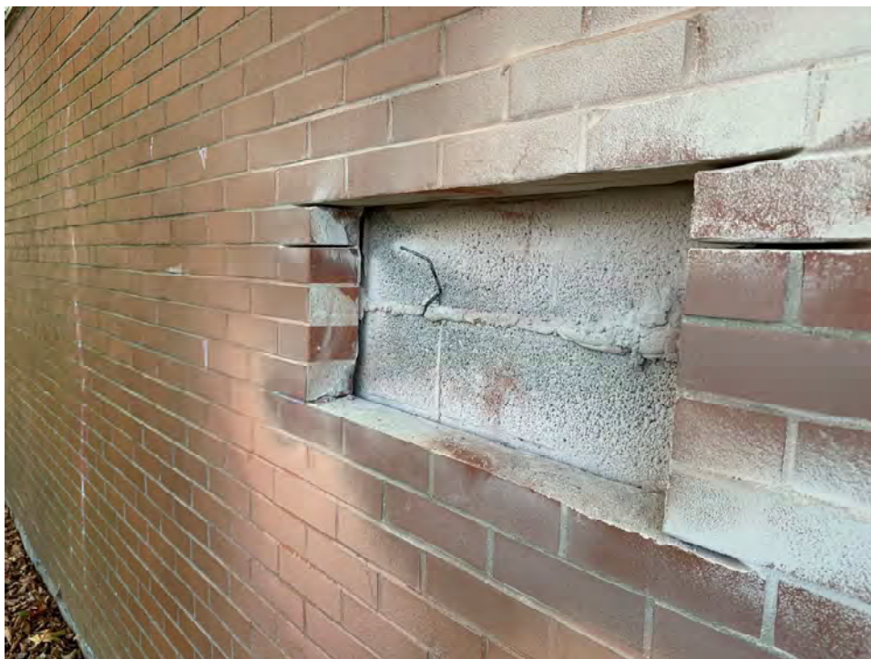
Photo 24: Exploratory brick opening on north elevation
