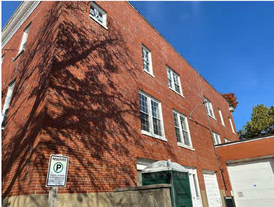
Photo 3: Overview of Old Fire Hall east elevation
