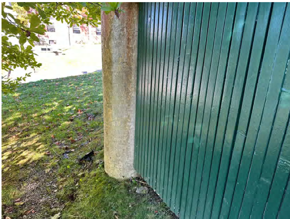
Photo 12: Concrete pier foundation and vertical trim below the Bandstand deck
