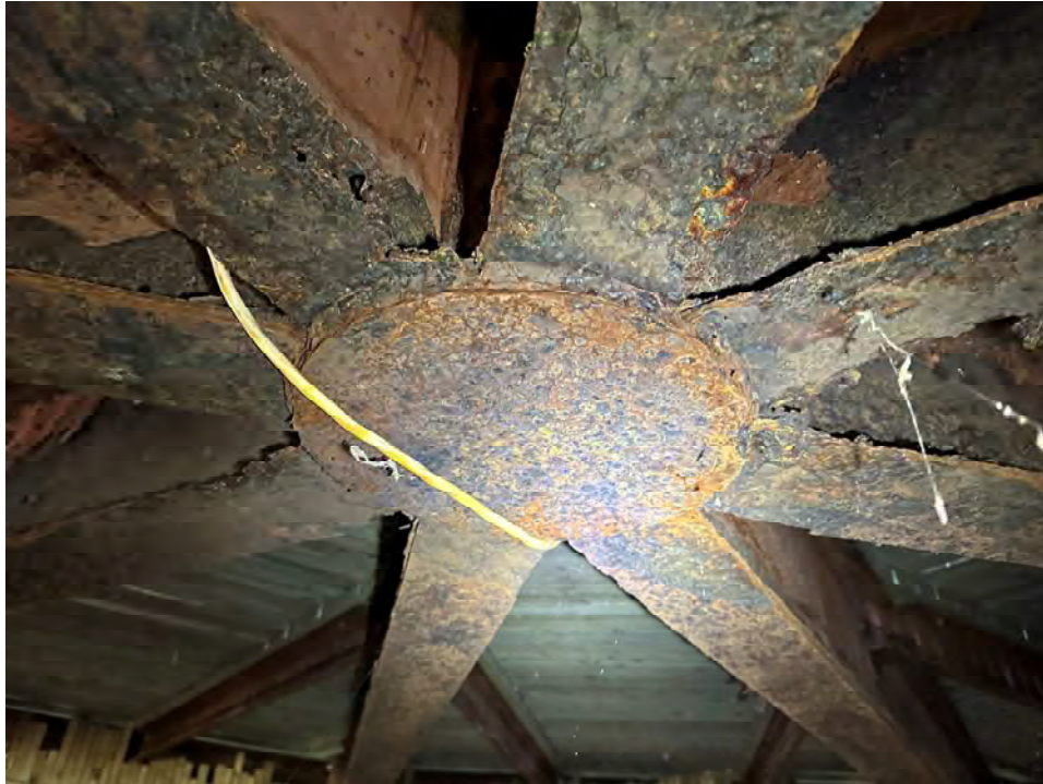
Photo 3: Underside of central point of deck's structural steel
