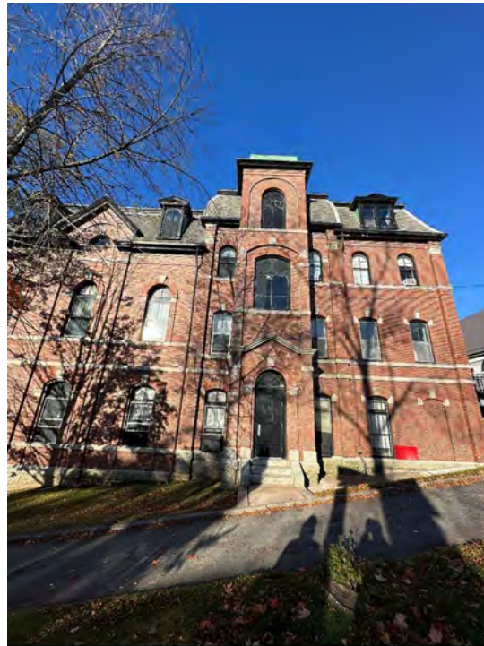
Photo 3: Overview of Town Hall east elevation
