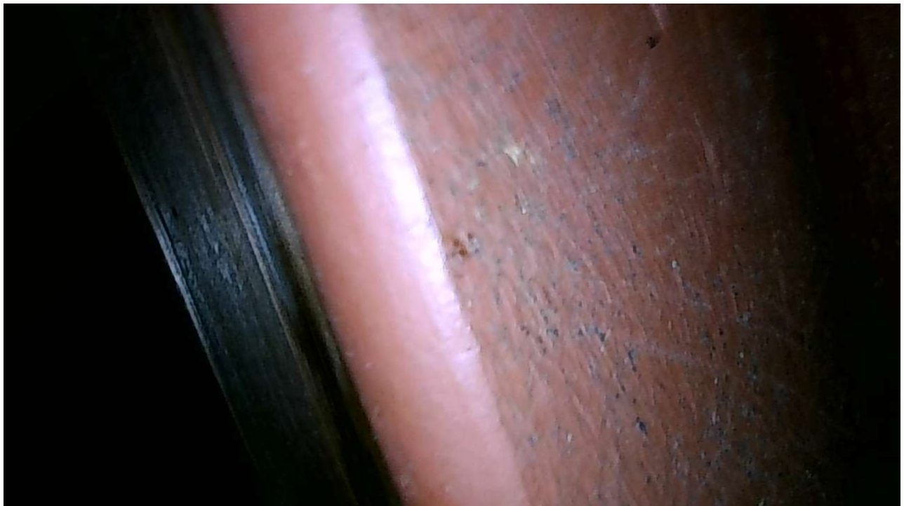
Photo 8: Borescope close-up image of roof steel beam flange
