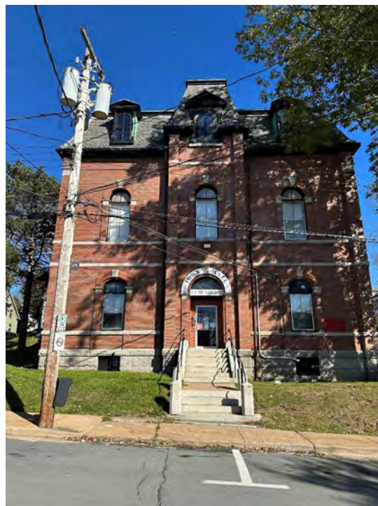
Photo 4: Overview of Town Hall south elevation (Cumberland Street Entrance)
