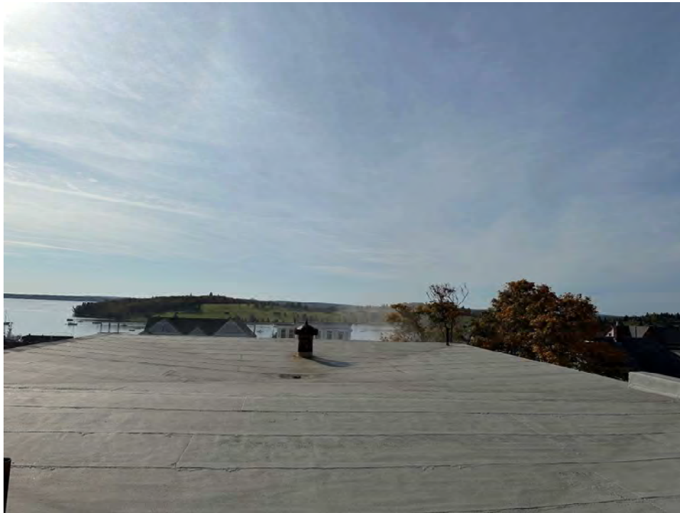
Photo 14: Overview of existing roofing membrane
