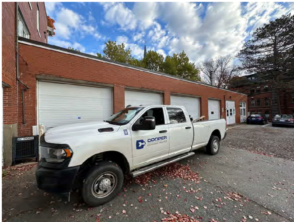
Photo 2: Overview of Electric Light Shop south elevation
