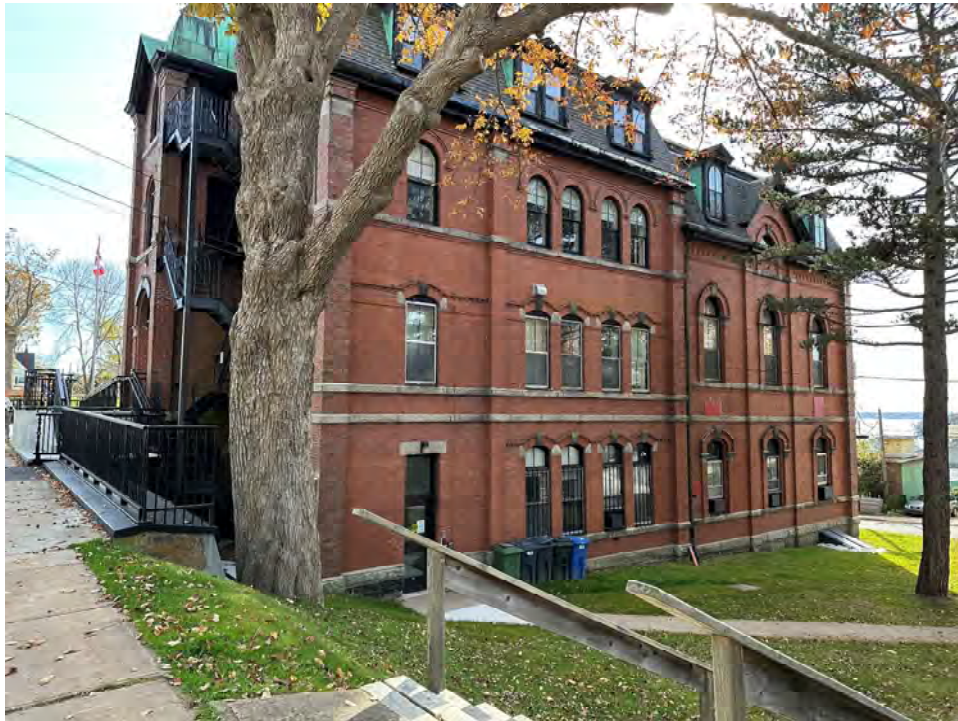
Photo 5: Overview of Town Hall west elevation
