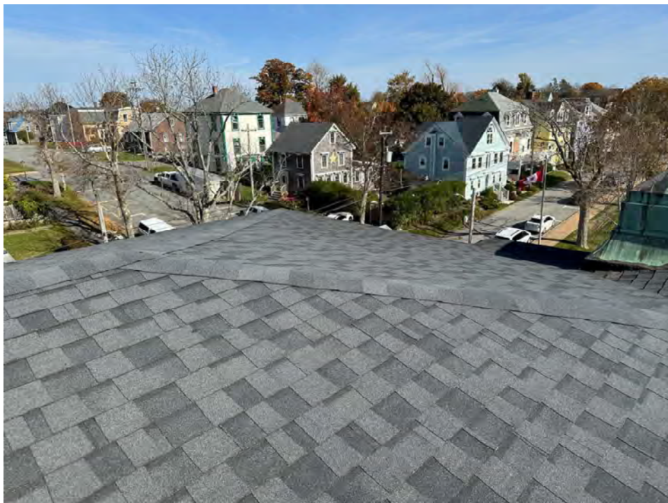
Photo 12: Newer asphalt shingles on north portion of roof
