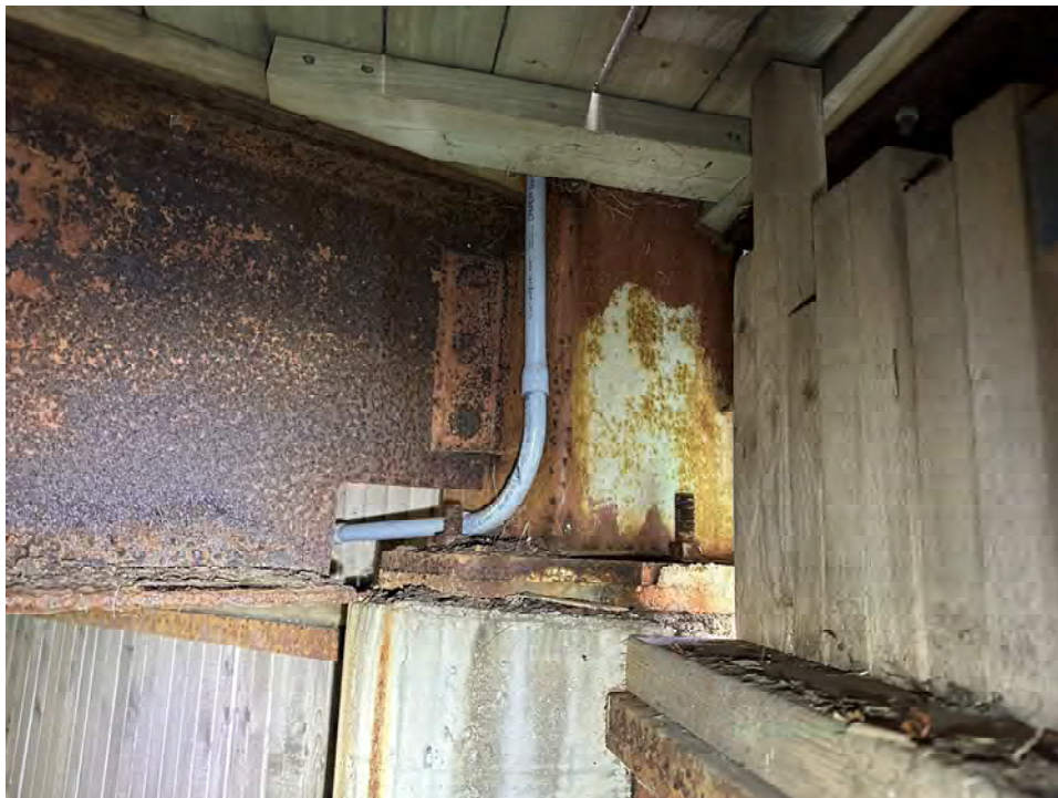
Photo 6: Structural steel beam to column connection (typ. at eight locations)
