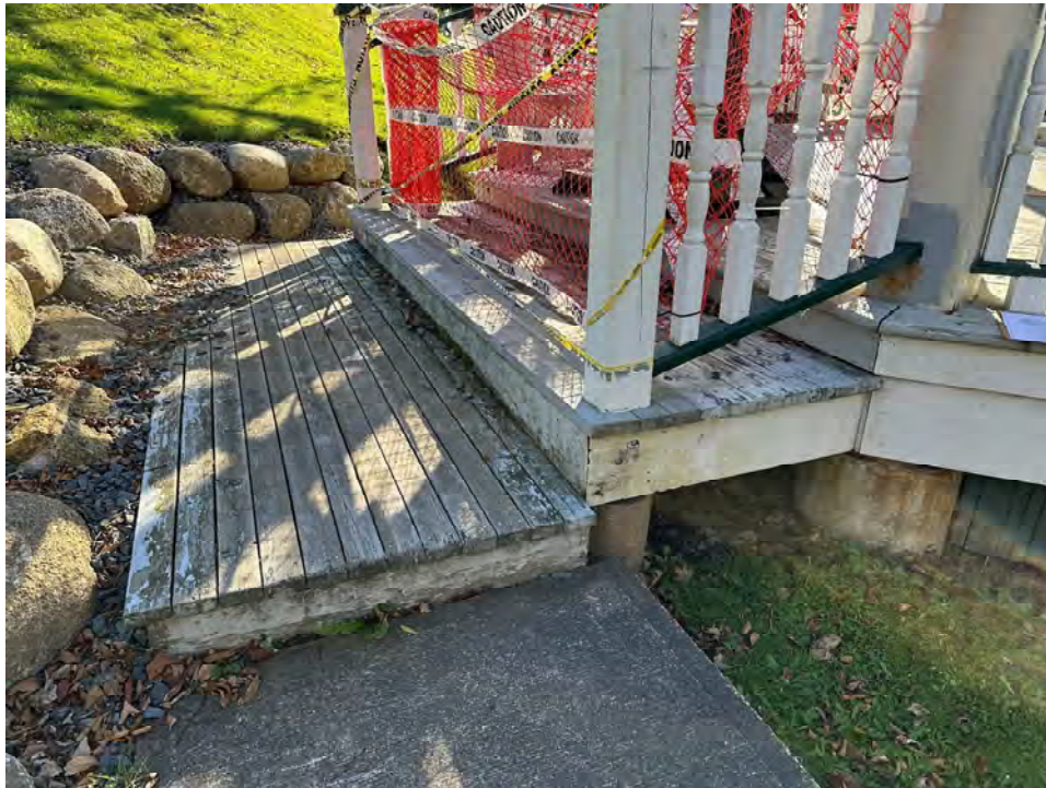
Photo 13: Access platforms on north side of Bandstand
