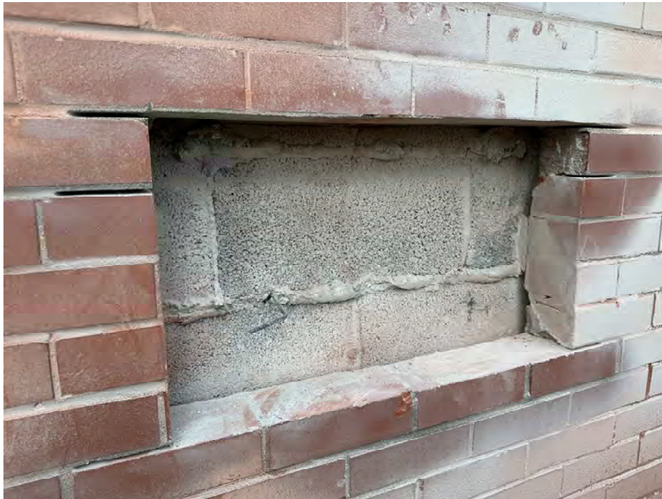
Photo 23: Exploratory brick opening on east elevation
