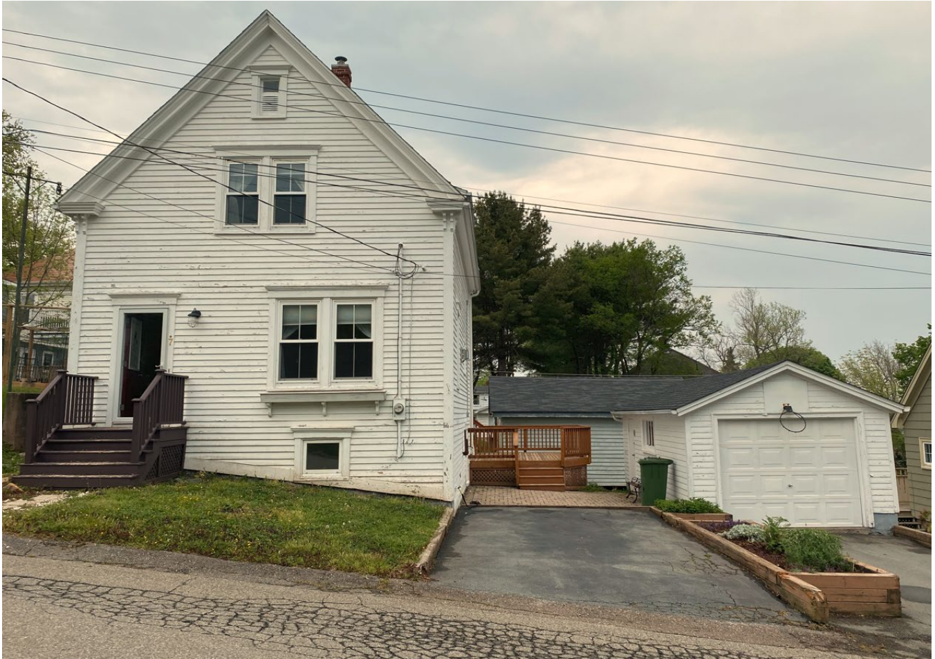
Attachment D – Photograph of Existing Pathway, Stairs and Driveways
