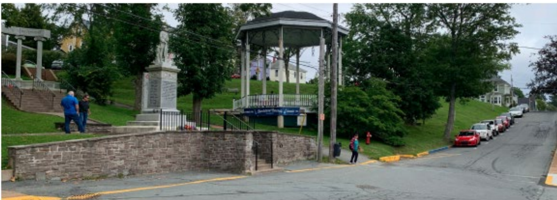
Image: Photo taken during the Design Team's initial site visit. View from Cumberland St.
