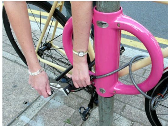
Example of Bike Rack Mounted on Sign or Parking Meter Pole
