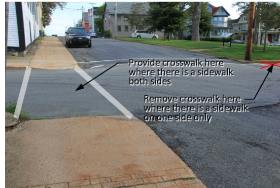
Example of Relocation of Crosswalk
