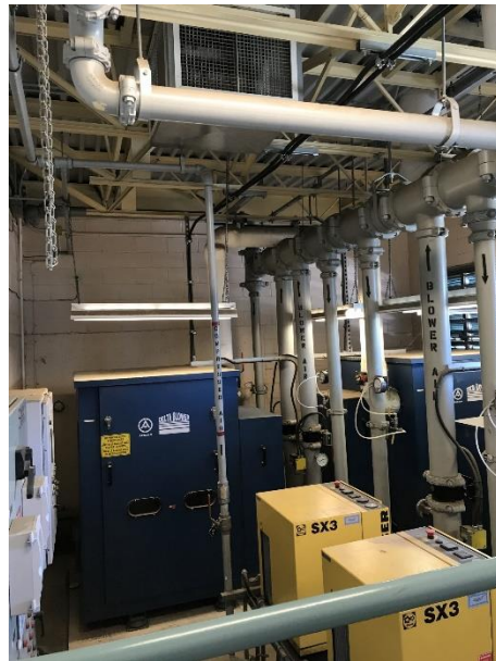
Figure 12 and 13: Existing Blower Room Layout and Louver
