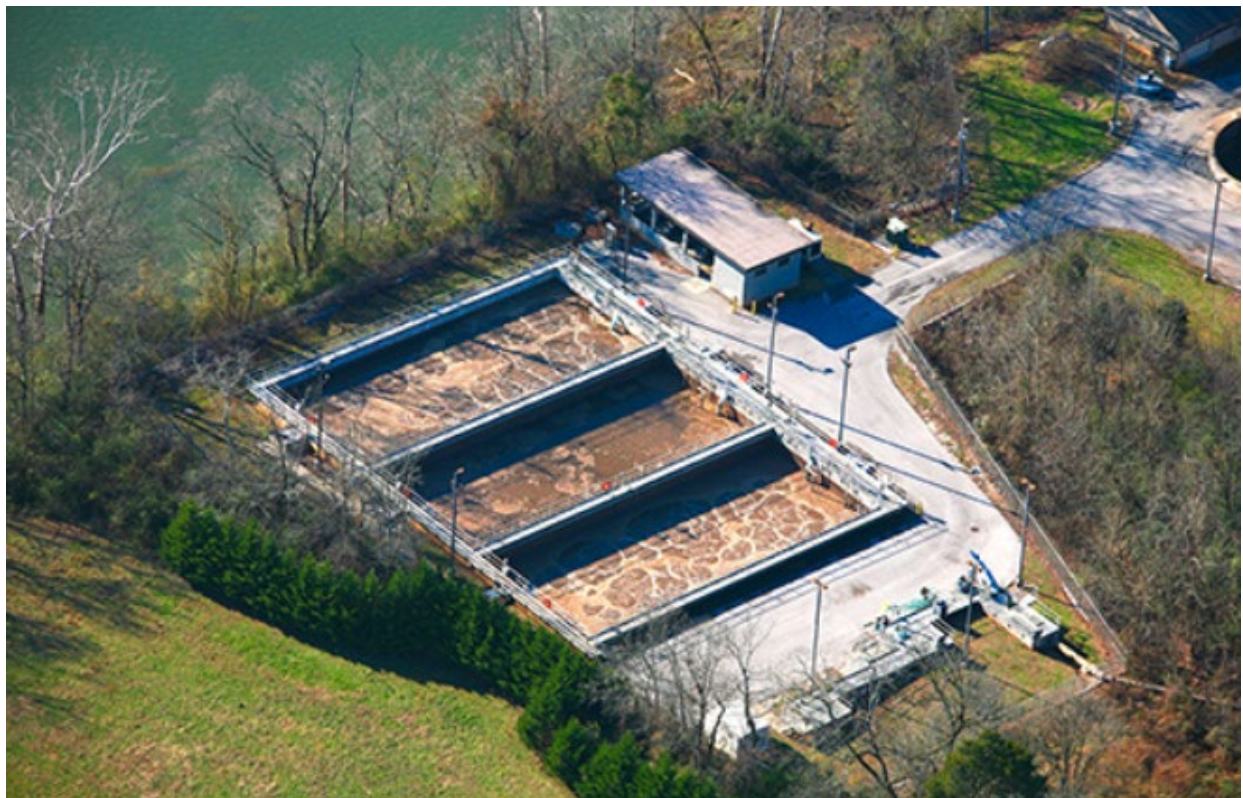
Figure 8: Installation of a three-train SBR system
