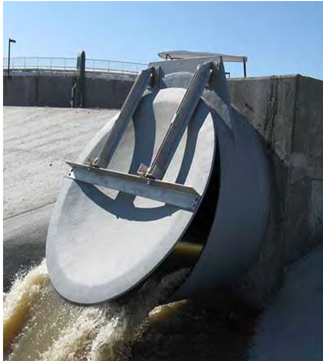
Gravity Type Flap Gate
