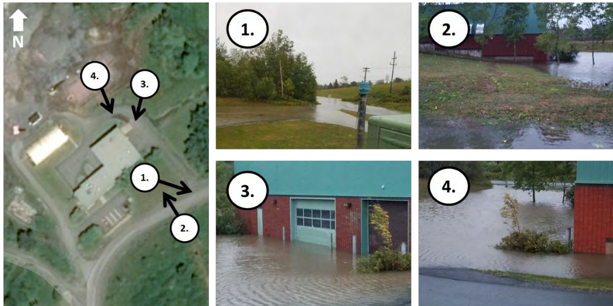
Figure 1-3: Flooding at the Lunenburg WWTP on September 7 th 2019
