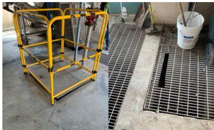
Figure 4: Existing Bilco Hatch to be replaced (left) and example of grating to be replaced (right)
