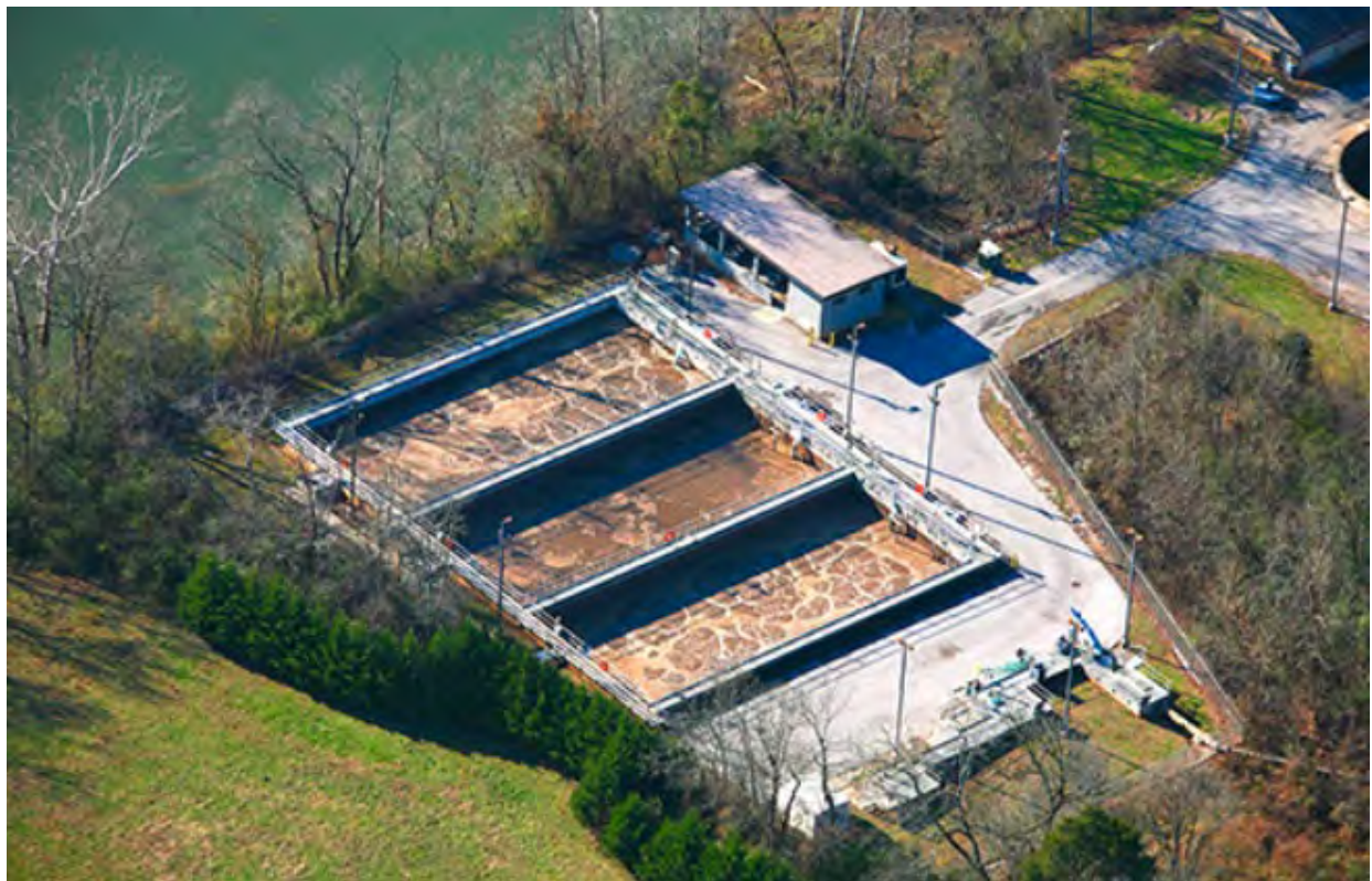
Figure 8: Installation of a three-train SBR system
