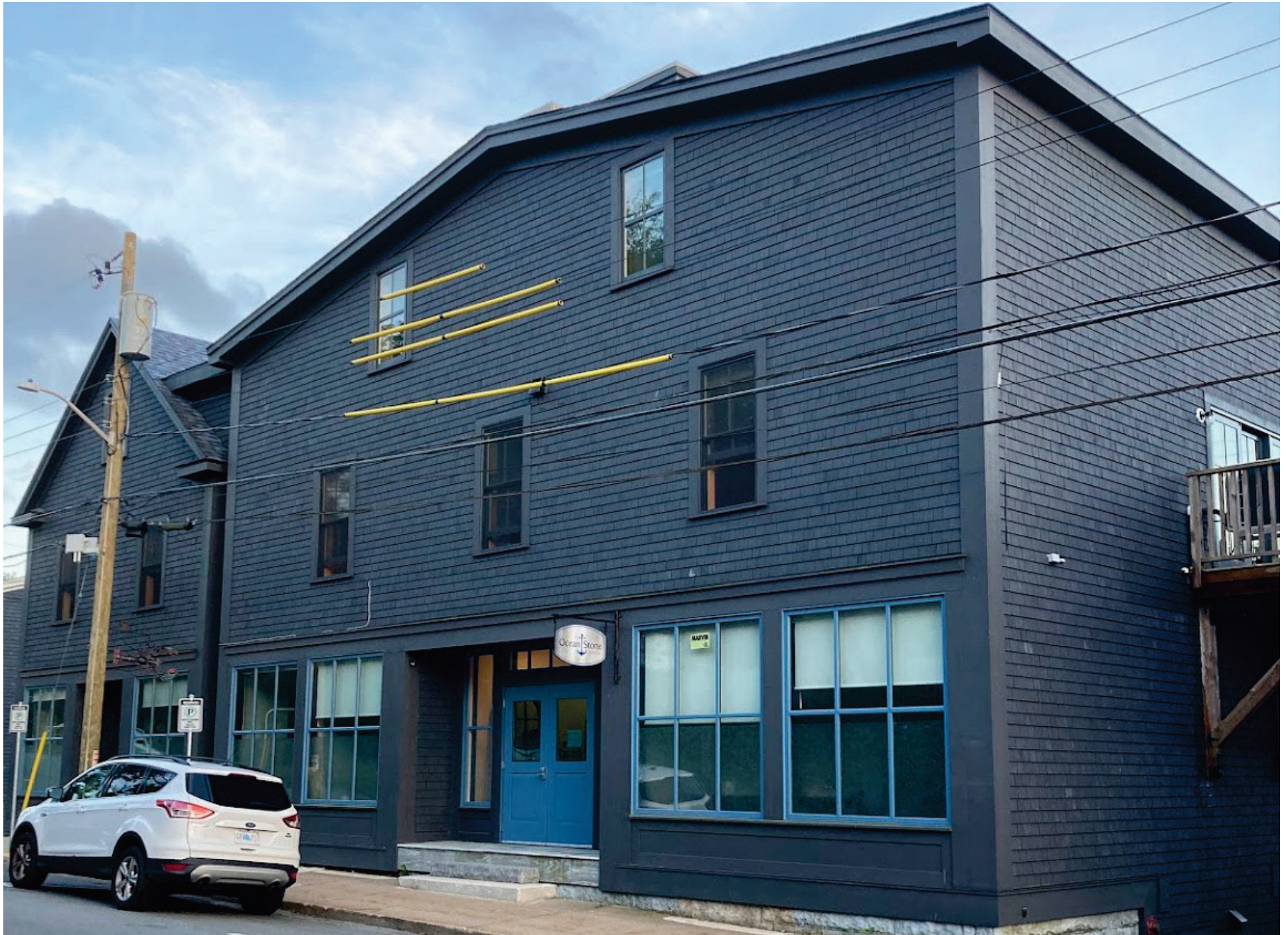
3 storey, symmetrical facade
