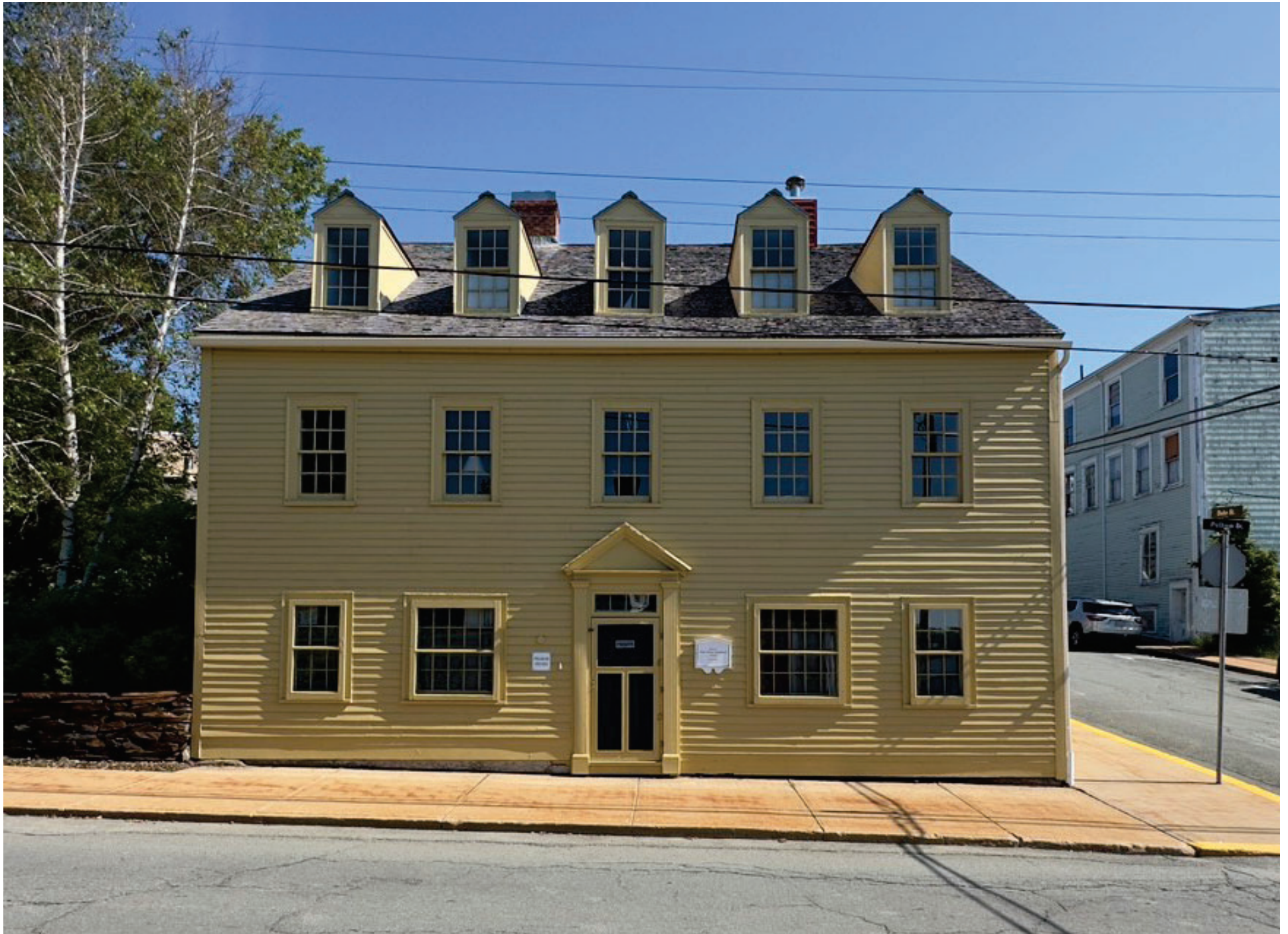
2 1/2 storey, symmetrical facade, dormers
