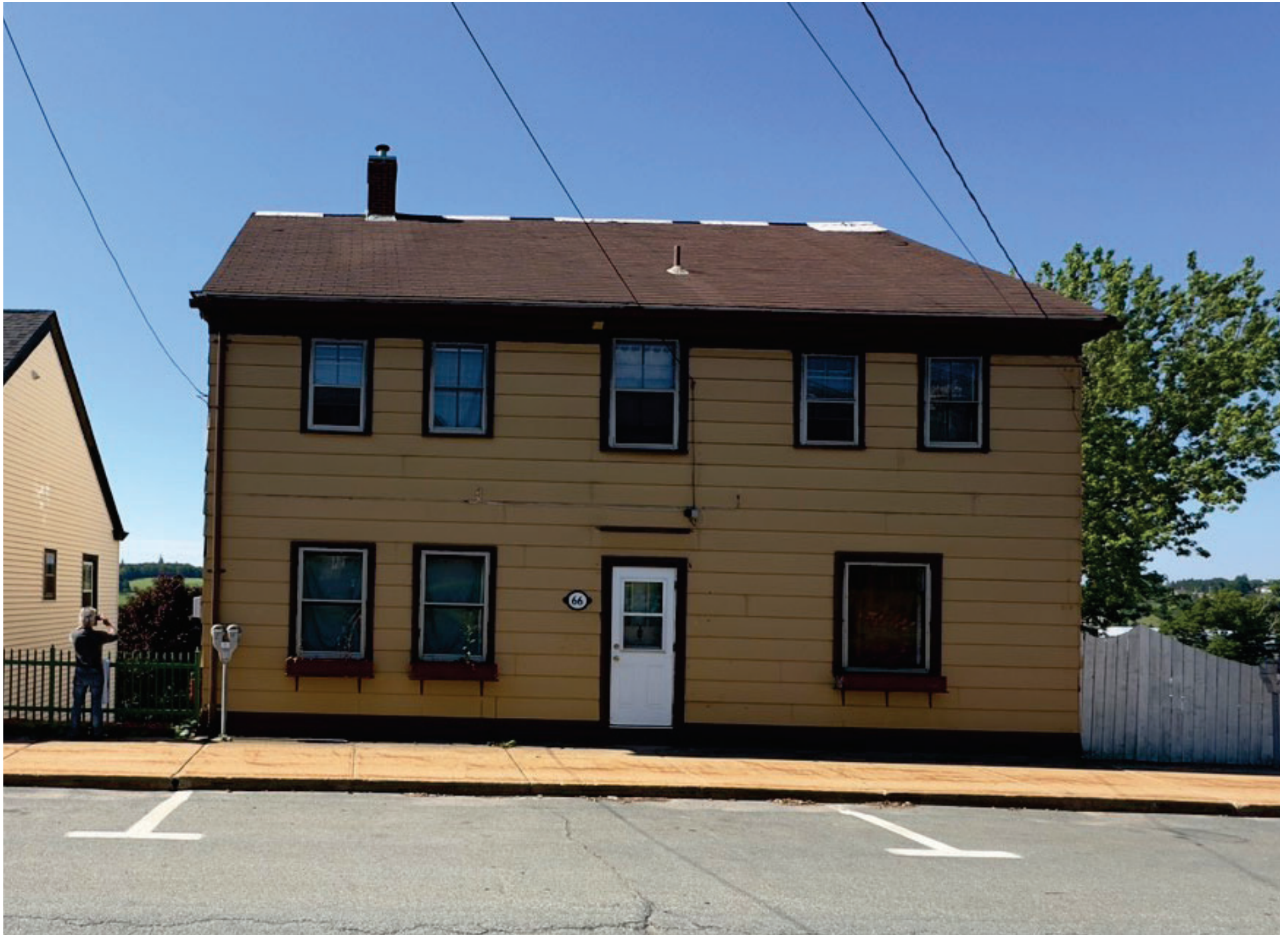
2 storey, asymmetrical facade
