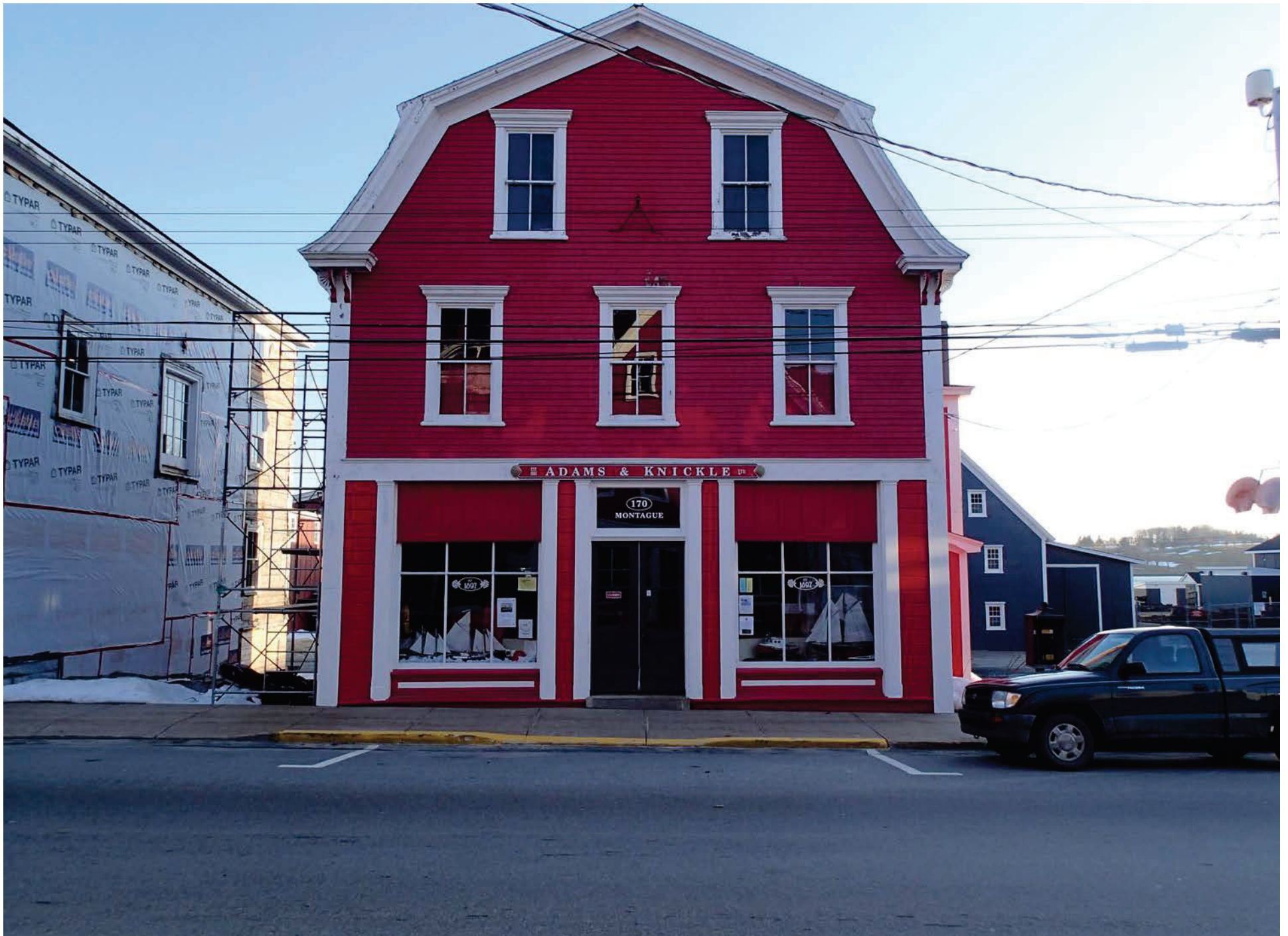
gambrel roof, shutters
