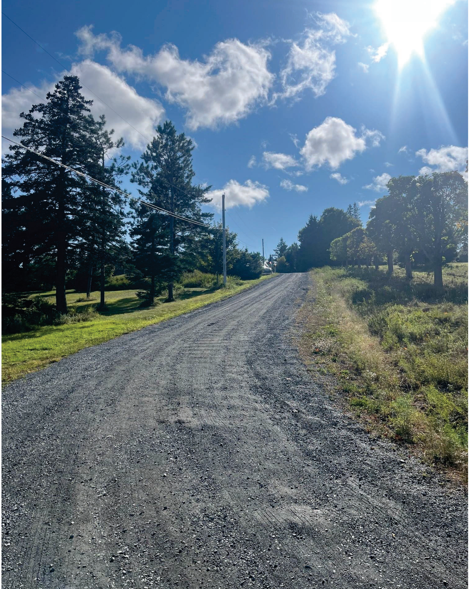
Knickle Road Ext. around bend at bottom of slope looking westerly
