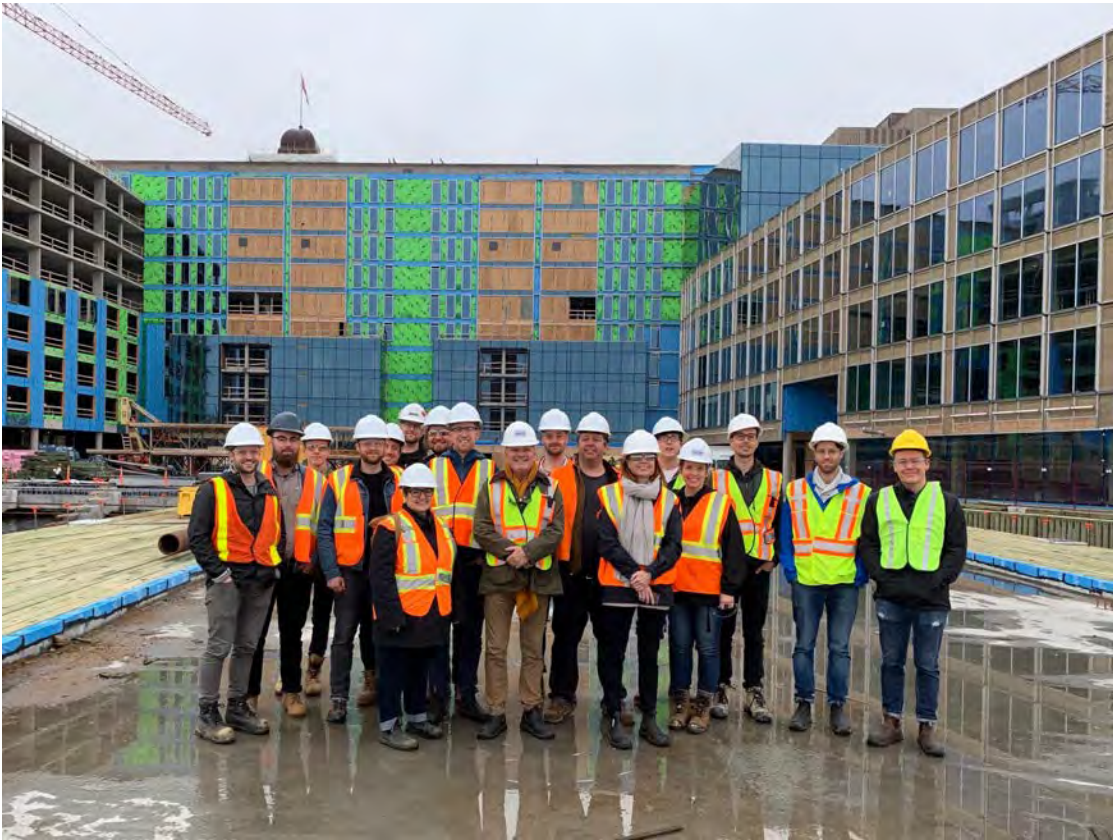
(top) MLSA team at Queen's Marquee during construction
