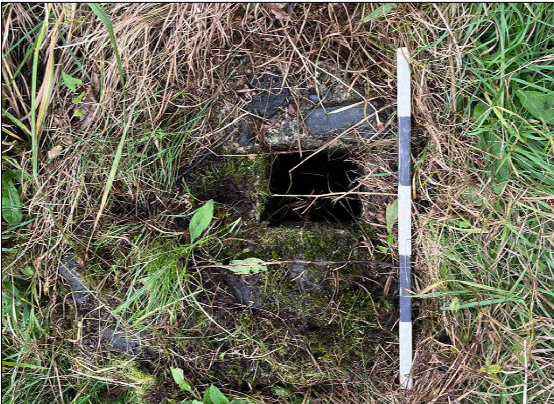
Plate 17: One of the concrete bases with a square hole in the tall grass surrounding Feature 1.
