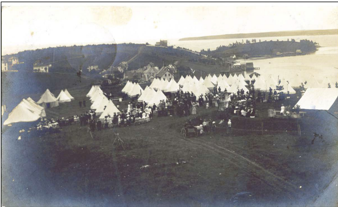
Figure 4-16: An undated photograph of Blockhouse Hill showing the berm (right), with young trees planted around the outside of it. Courtesy Ralph Getson via Henry Cary.
