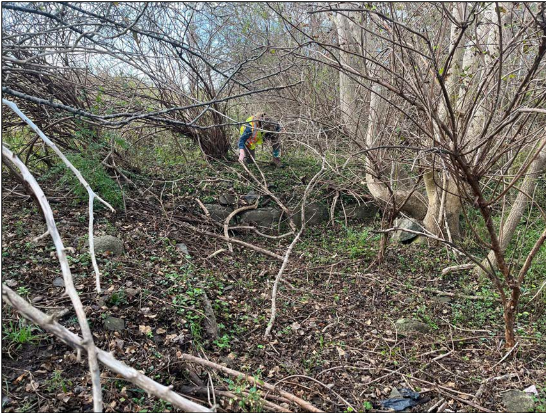
Plate 13: Feature 1, a concrete and stone foundation belonging to the former Lunenburg County Jail, facing south.
