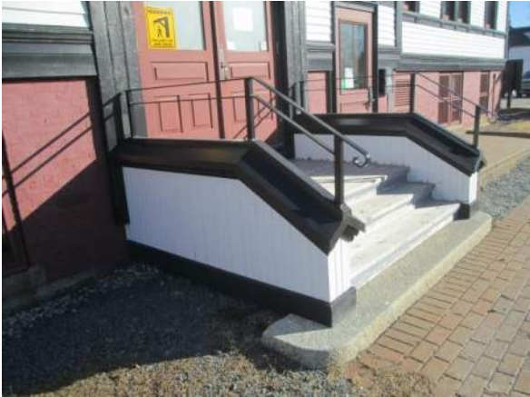
Figure 39 – Stair rebuilt in 2016 and guardrails installed in 2018 – good condition.
