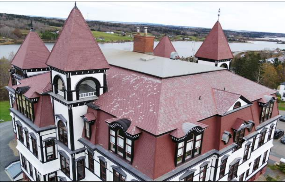
Figure 51 – West-South Elevation. Overall view
