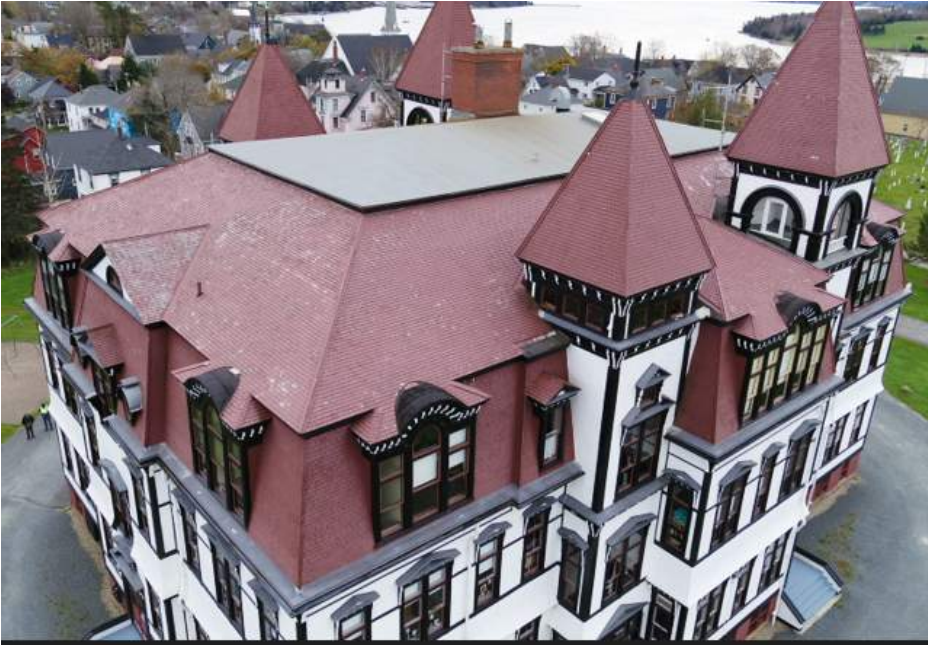
Figure 50 – North-West Elevation. Overall view
