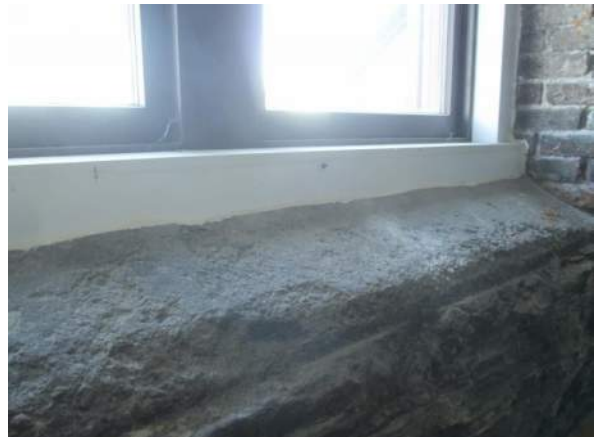
Figure 80 Stone sill with new windows installed in 2018. Also see photo 32.
