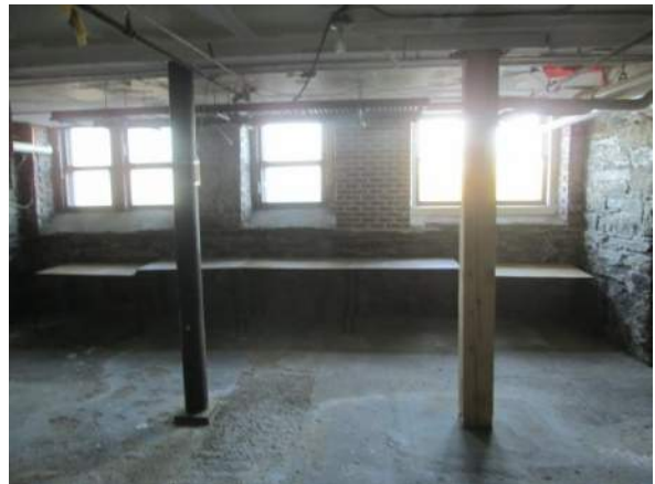
Figure 78 – Room B24: looking West.
