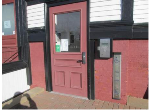
Figure 42 – New door in 2020 and new door operator panel.
