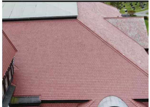
Figure 68 – East Elevation (left side). The Roof condition is satisfactory.
