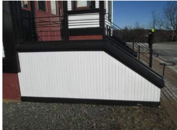
Figure 5 – LHS entry stair rebuilt in 2017 – good condition.
