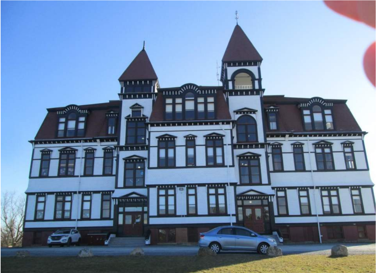
Figure 27 – West Elevation: Envelope restoration work completed in 2018. (does not include brick foundation wall)
