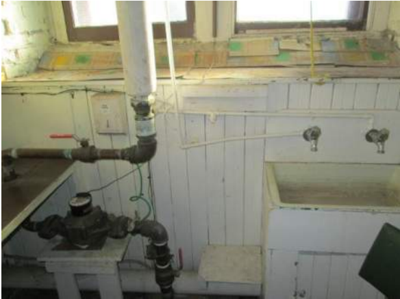
Figure 91 – Room B26 wood sill and knee-wall built over stone foundation wall.
