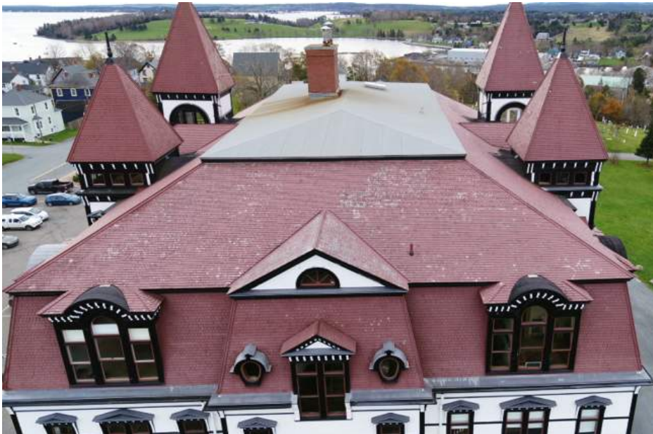
Figure 49 – North Elevation. Overall view
