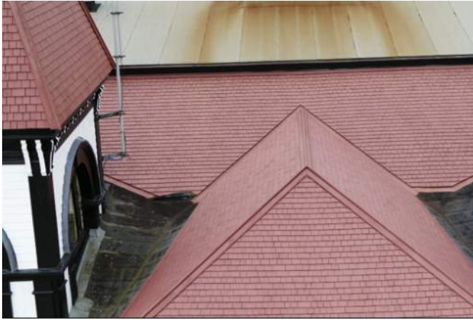
Figure 67 – East Elevation (center). The Roof condition is satisfactory.
