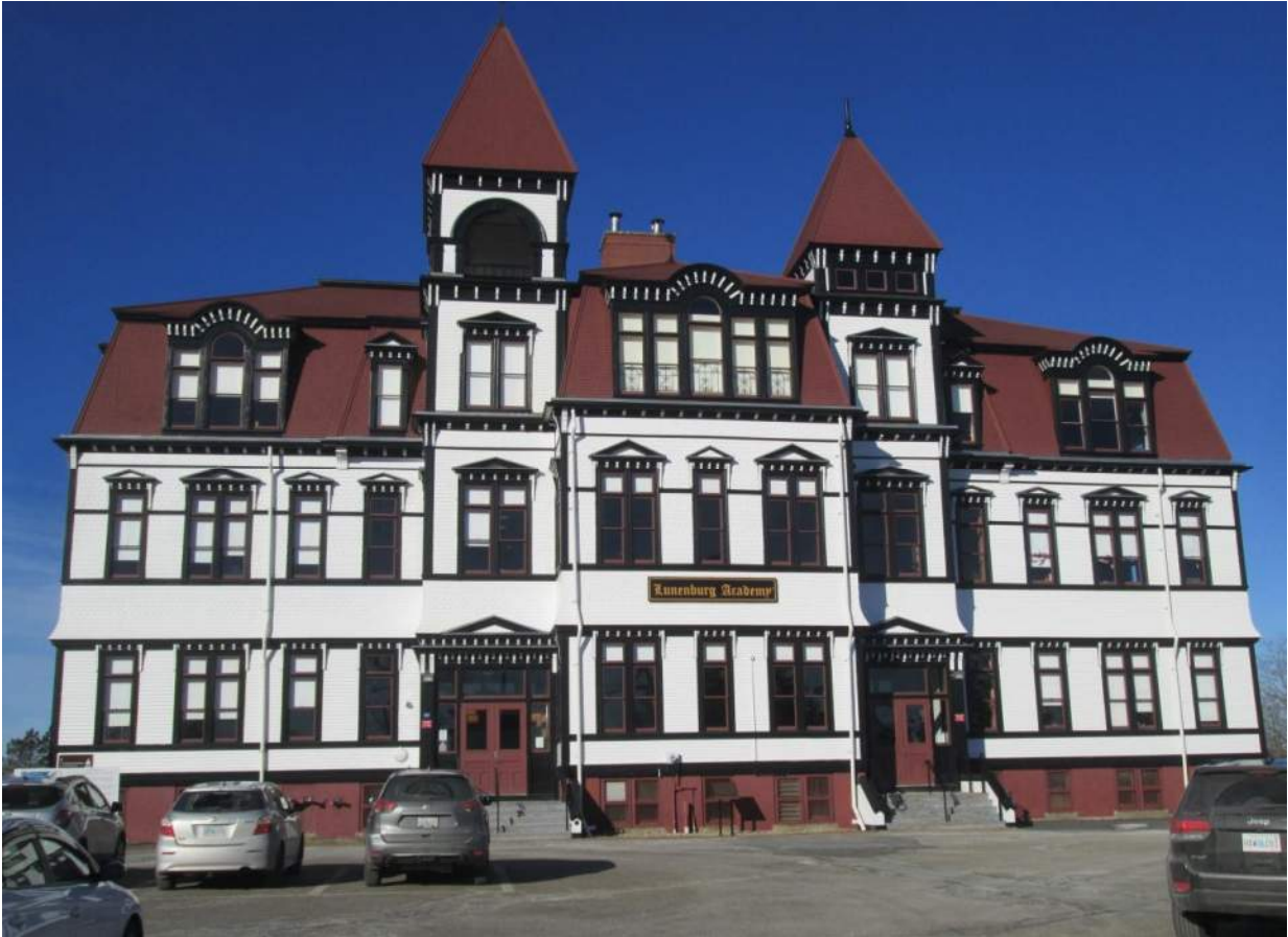
Figure 1 – East Elevation: Envelope restoration work completed in 2020. (does not include brick foundation wall)
