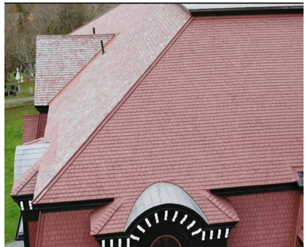
Figure 66 – East Elevation (left side). The Roof condition is satisfactory."
