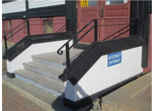
Figure 40 Stair rebuilt in 2016 and guardrails installed in 2018 – good condition.
