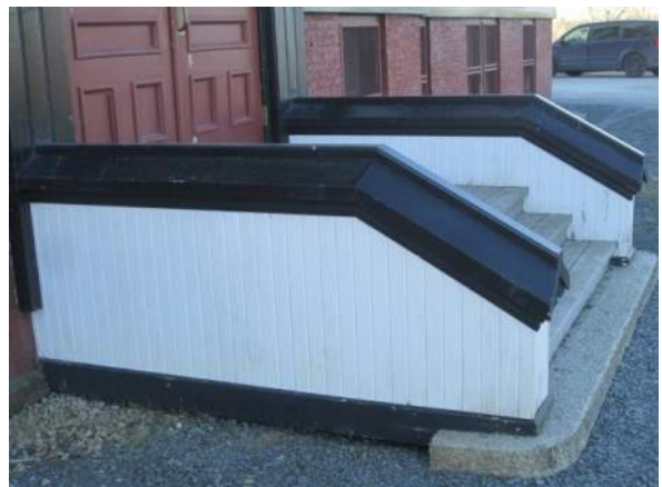
Figure 17 – Stairs to North doors rebuilt in 2016 - good condition.
