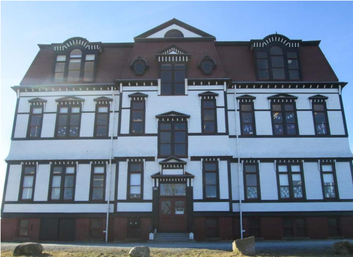
Figure 15 – North Elevation: Envelope restoration work completed in 2018. (does not include brick foundation wall)
