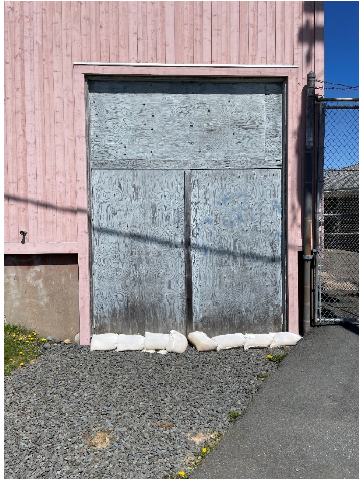
Photo 2. Existing South Side Wooden Doors
