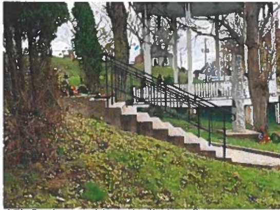
15) Stairs and handrails leading to cenotaph
