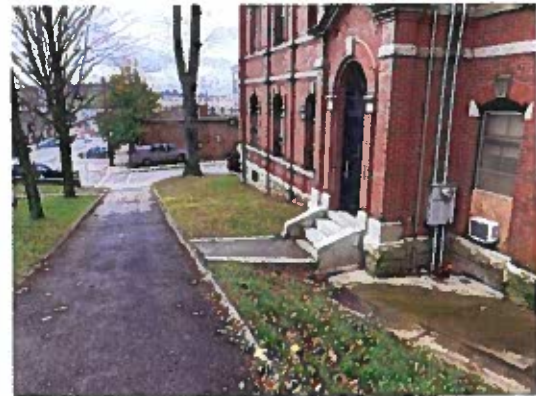
10) Pathway along east side of Town Hall
