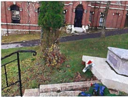
19) Handrail termination at cenotaph
