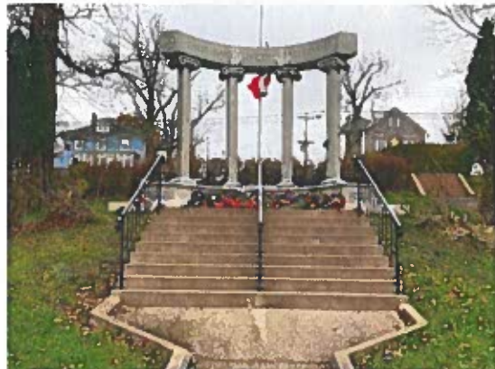
16) Stairs and handrails leading to cenotaph
