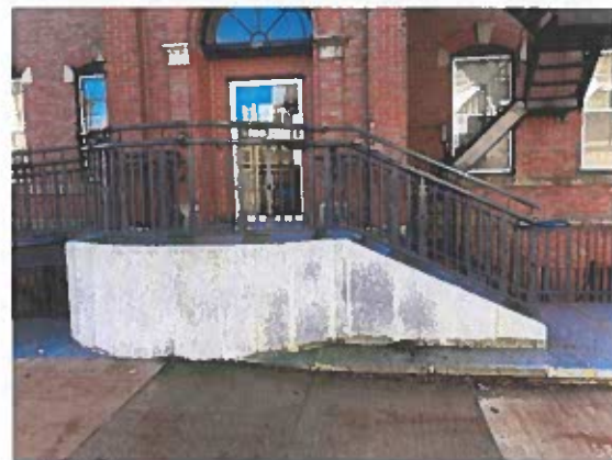
6) Stair and ramp at Town Hall Townsend Street entrance
