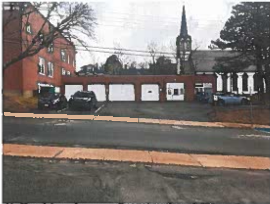
1) Parking lot on Cumberland Street east of the Fire Hall
