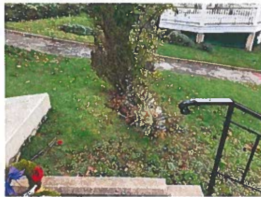
18) Handrail termination at cenotaph
