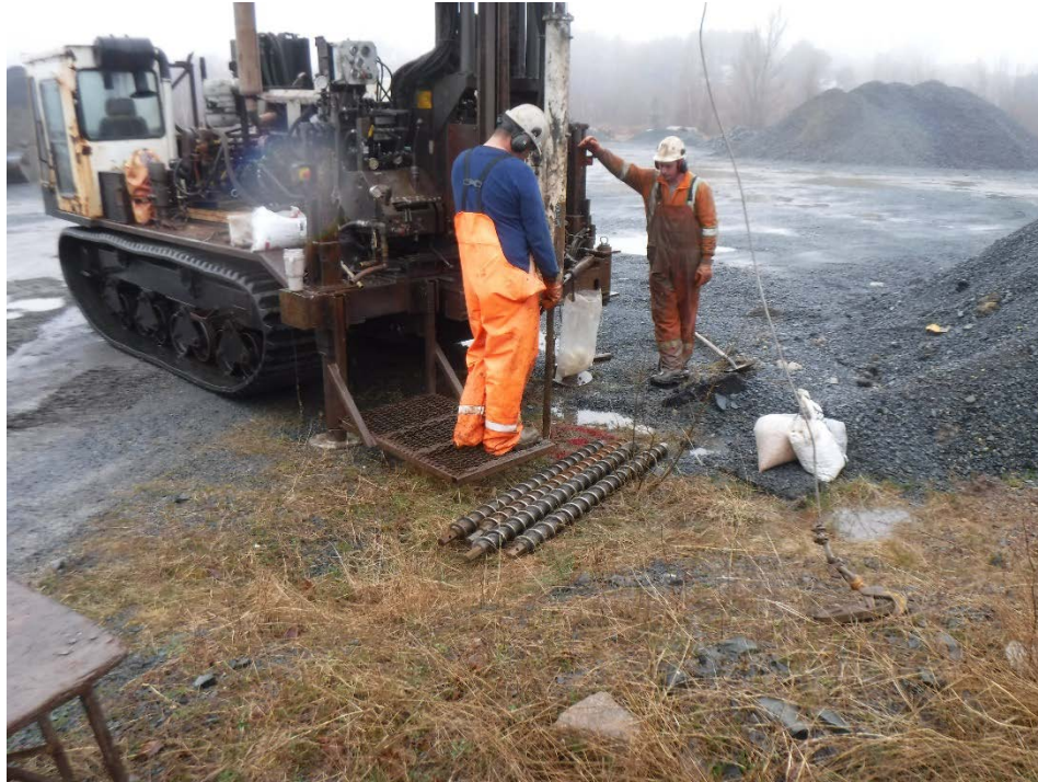
Photo 1: Drilling 24MW02, looking north.
