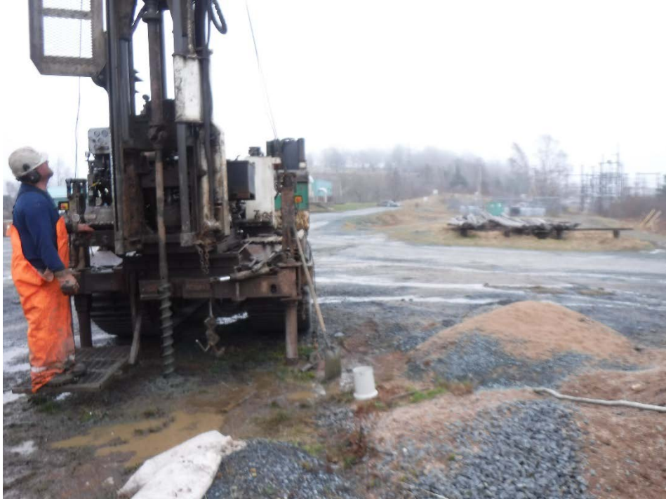
Photo 3: Drilling 24MW05, looking south.
