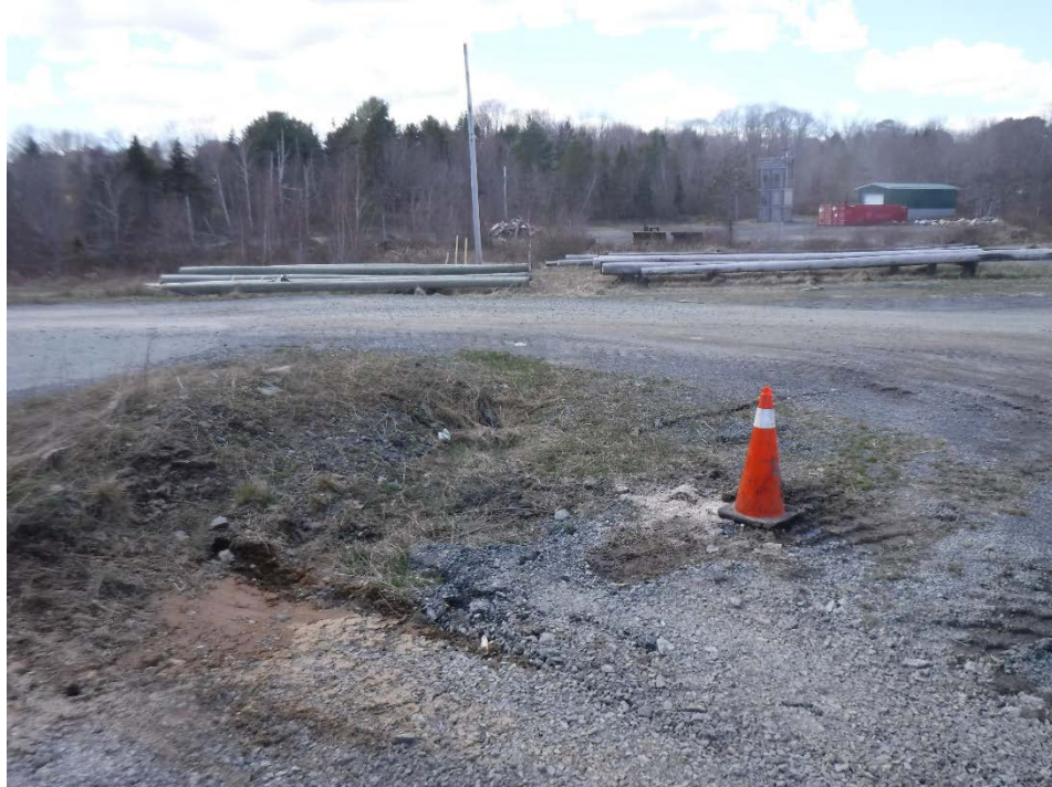
Photo 5: View of 24MW02, adjacent to cone. Looking southwest
