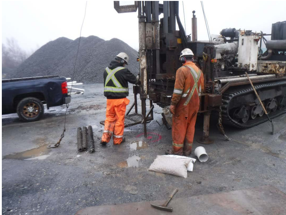
Photo 2: Drilling 24MW03, looking west.
