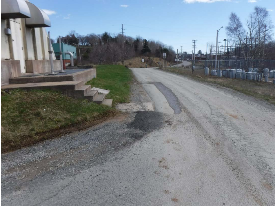
Photo 11: View of south entry driveway, looking southeast.
