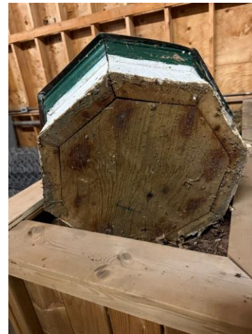
Photos 1,2,3: Existing roof ornament for repair re-attachment
