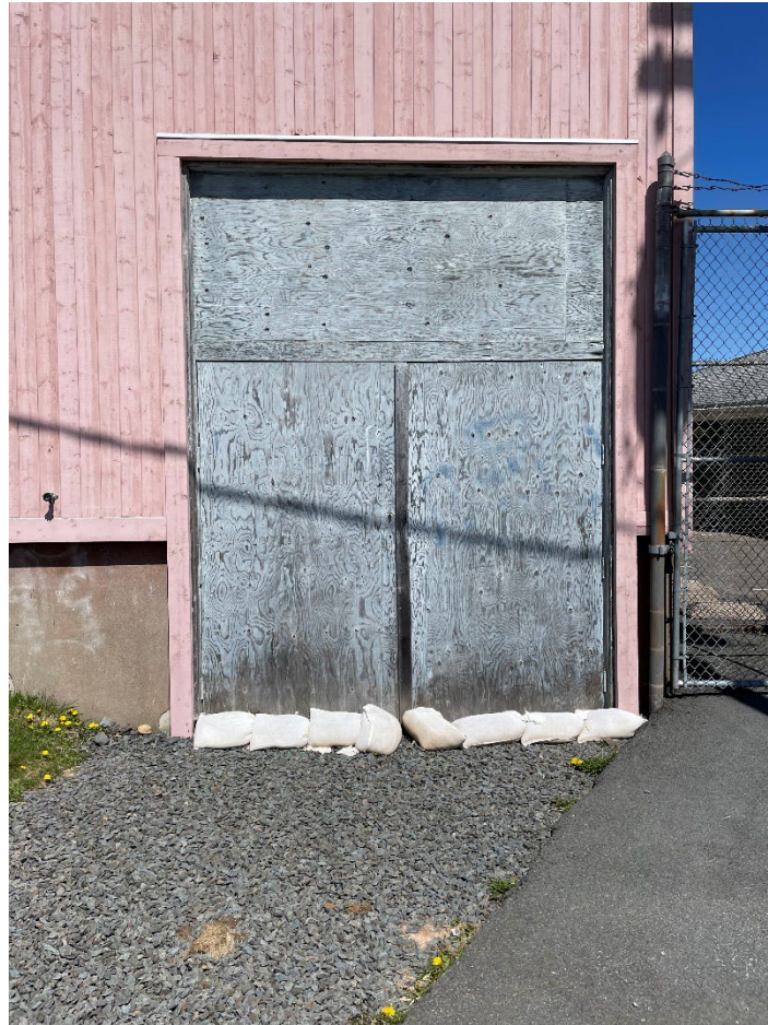
Photo 2. Existing South Side Wooden Doors
