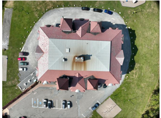
General Overhead – Mod. Bit.
