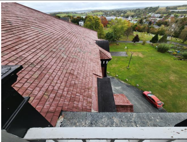
View from tower looking towards eye-brow dormer
