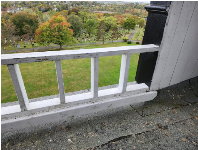
General – Existing Railing, Mod. Bit. at tower
