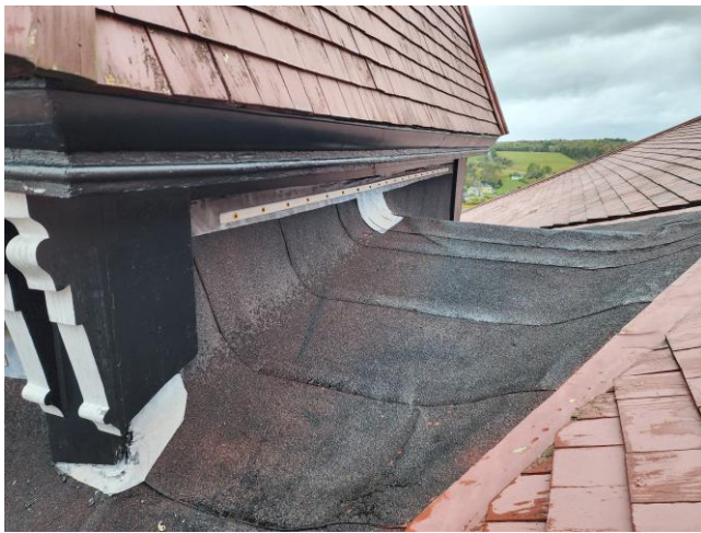
General – Existing saddle at backside of tower
