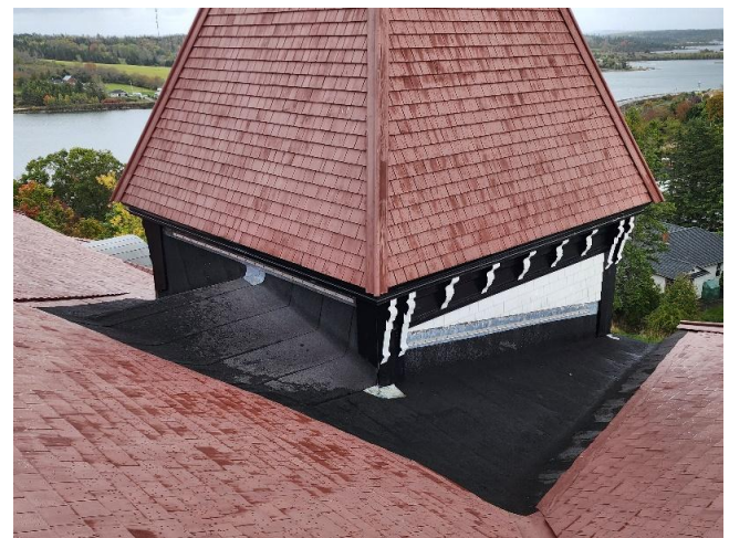
General – Mod. Bit. at Towers
