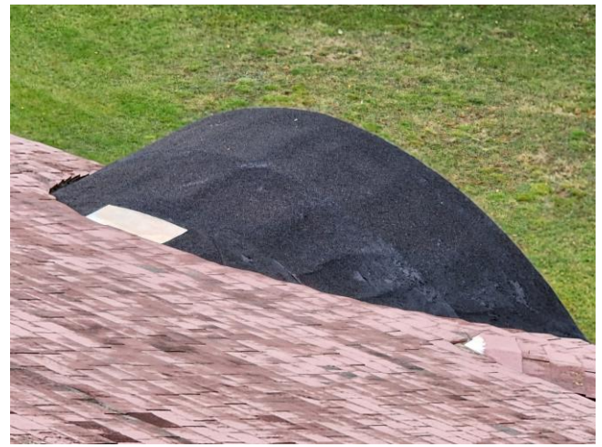
General – existing conditions – eyebrow dormer
