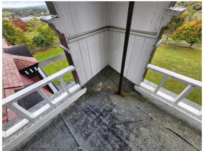
General – existing mod. bit., penetration at tower
