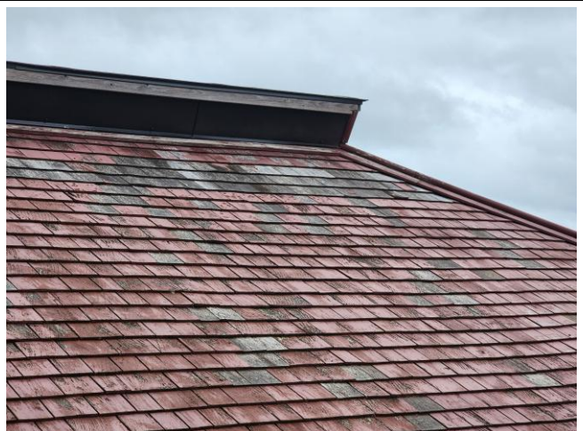
General – Existing condition at fascia below mod. bit.
