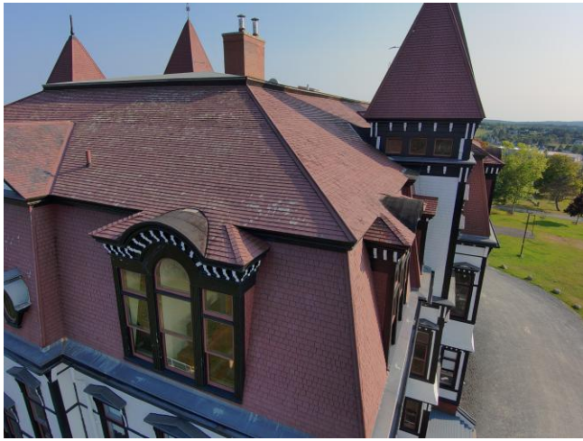
General – Sloped roof area and eye-brow dormer
