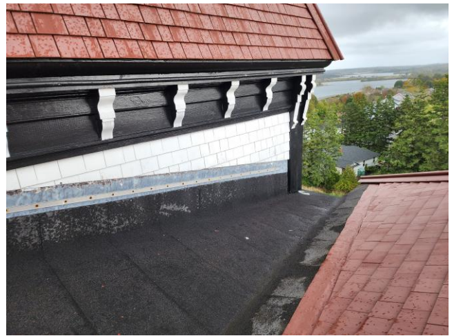
Existing – mod. bit. at sidewall of tower
