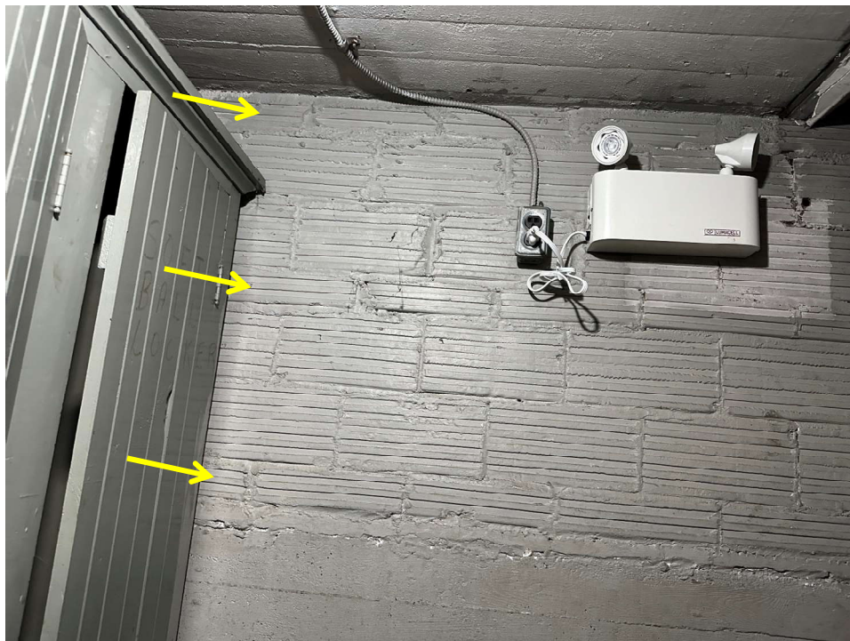
Photo 7: Structural clay tile as visible from building basement. Yellow arrows at on bed courses
