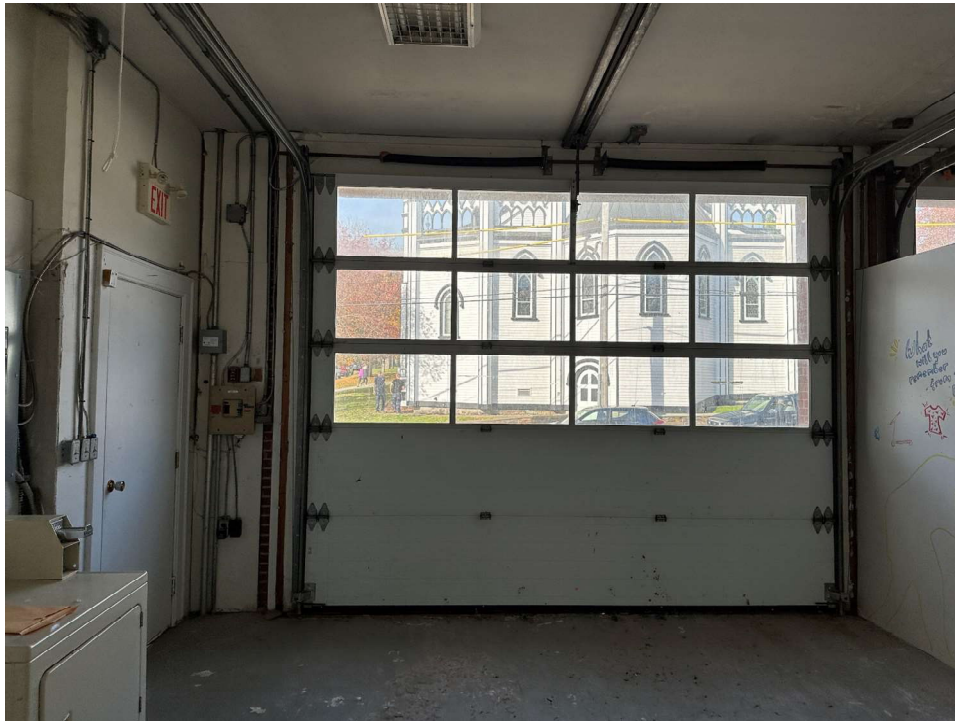
Photo 8: West elevation bay door interior (one of four)
