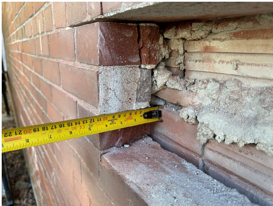
Photo 18: Exploratory brick opening on north elevation
