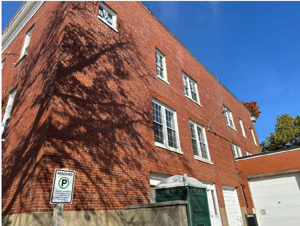
Photo 3: Overview of Old Fire Hall east elevation
