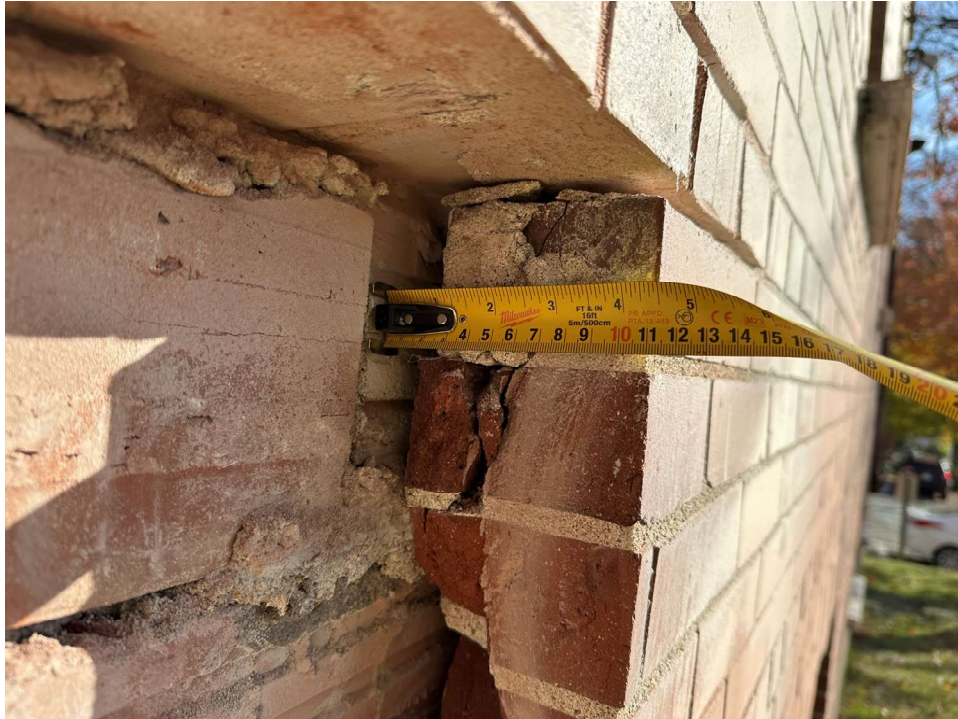
Photo 19: Exploratory brick opening on south elevation
