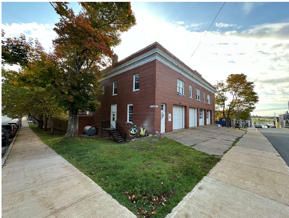
Photo 2: Overview of Old Fire Hall north and west elevation
