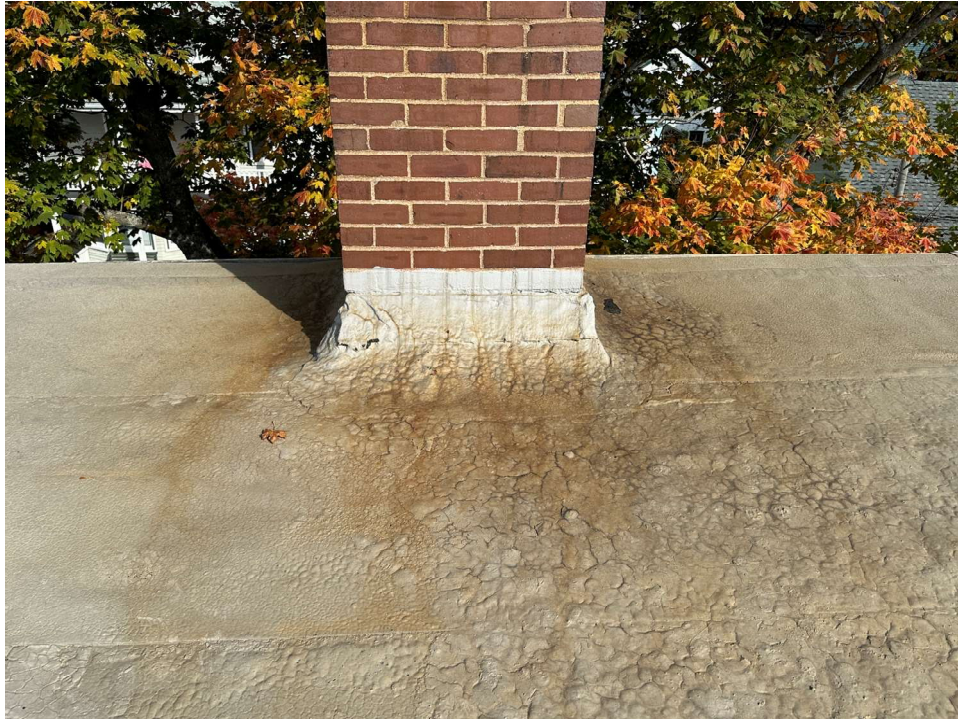
Photo 16: Alligator cracking on roofing membrane telescoping through the coating at north chimney
