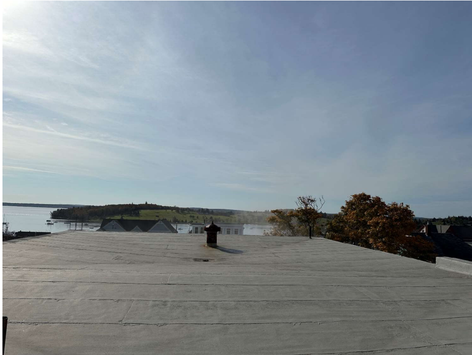
Photo 14: Overview of existing roofing membrane
