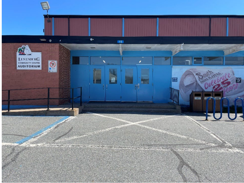
Photo 1. Existing Main Entrance
