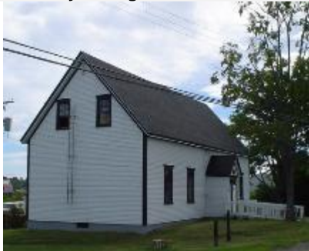
Front and North West Facades
