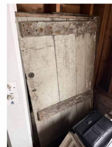
INTERIOR OF ORIGINAL DOOR
