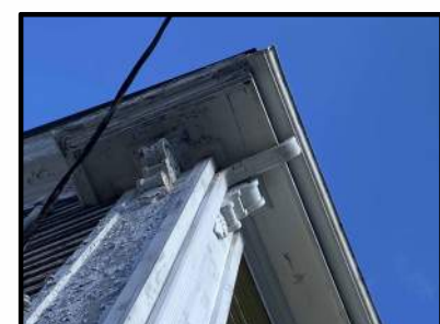
EXISTING CONDITION: STYLE OF KNAUT RHULAND HOUSE, SHOWING STYLE ALUMINUM GUTTER AND DOWNSPOUT ASSEMBLY.
