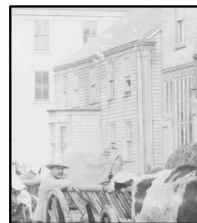
PRECEDENCE: CONTEXT: IMAGE OF HOUSE ON MONTAGUE STREET, LUNENBURG TOWN, 1980 SHOWING AN INTEGRAL GUTTER SYSTEM AND METAL DOWNSPOUT.
