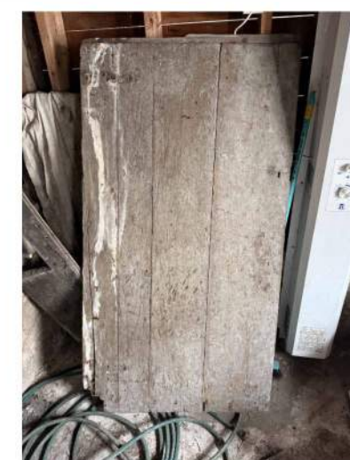
EXTERIOR OF ORIGINAL DOOR
