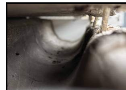
EVIDENCE: LENGTH OF EXTANT INTEGRAL GUTTER IN THE EAVE RETURN OF THE KNAUT RHULAND HOUSE.
