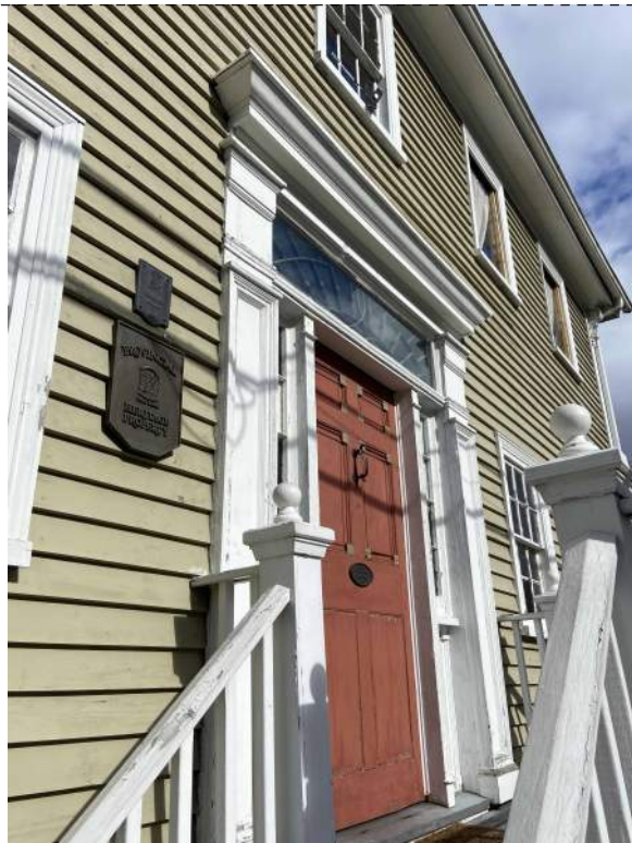
SOUTH (FRONT) DOOR
