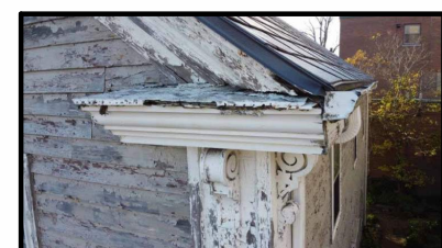
EXISTING CONDITION: THE SCROLLED FASCIA OF THE EAVE RETURN, AND LACK OF MATCHING FASCIA ON THE REAR OF THE KNAUT RHULAND HOUSE, EVIDENCE SUGGESTS THAT THE AREA OF THE GUTTER WHERE THE INTEGRAL GUTTER WOULD LOCATE, WAS REMOVED, ALONG WITH THE DECORATIVE FASCIA TRIM, AND REPLACED WITH A FLAT BOARD, TO MAKE A SUBSTRATE FOR THE S STYLE GUTTER, THEREBY SHORTENING THE DEPTH OF THE ROOF OVERHANG.
