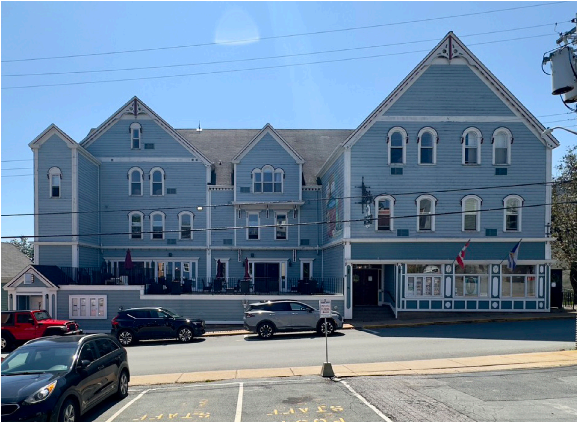
3 1/2 storey, asymmetrical facade
