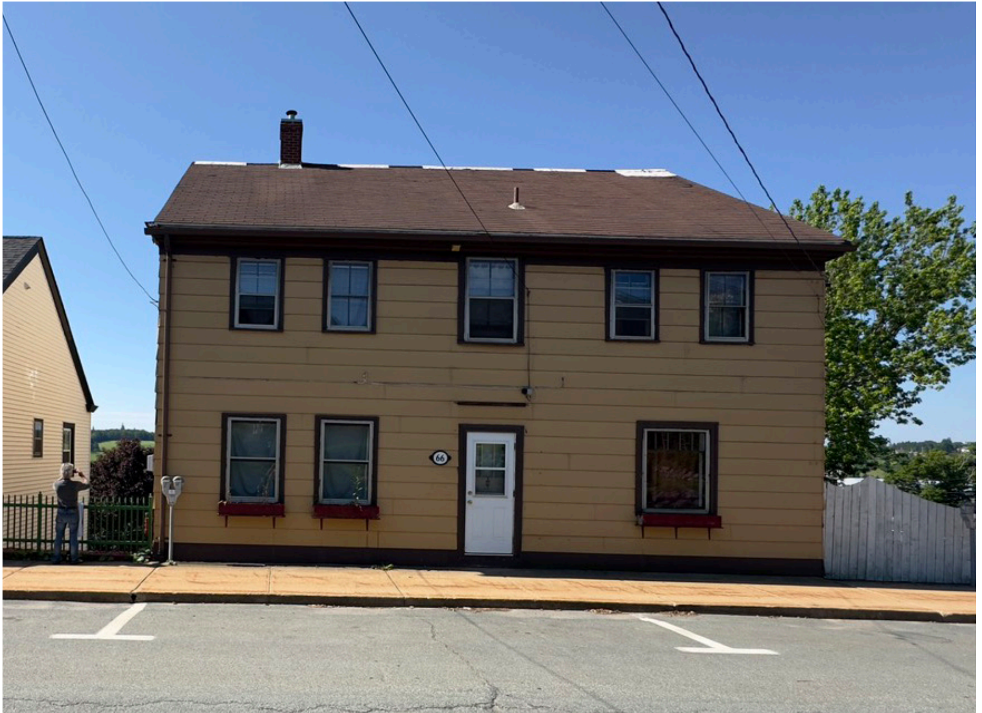
2 storey, asymmetrical facade
