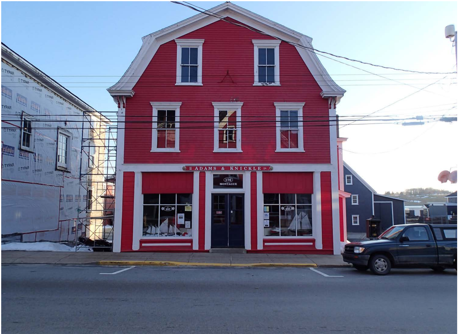
gambrel roof, shutters
