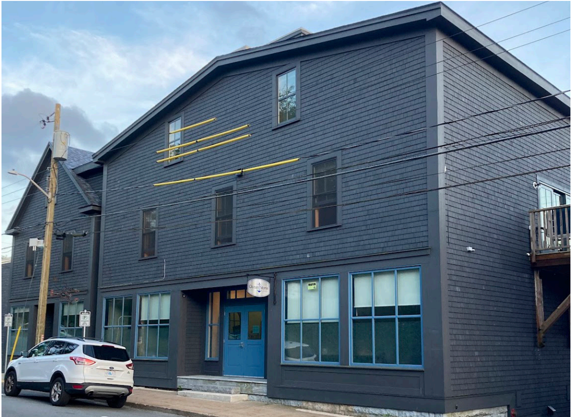
3 storey, symmetrical facade
