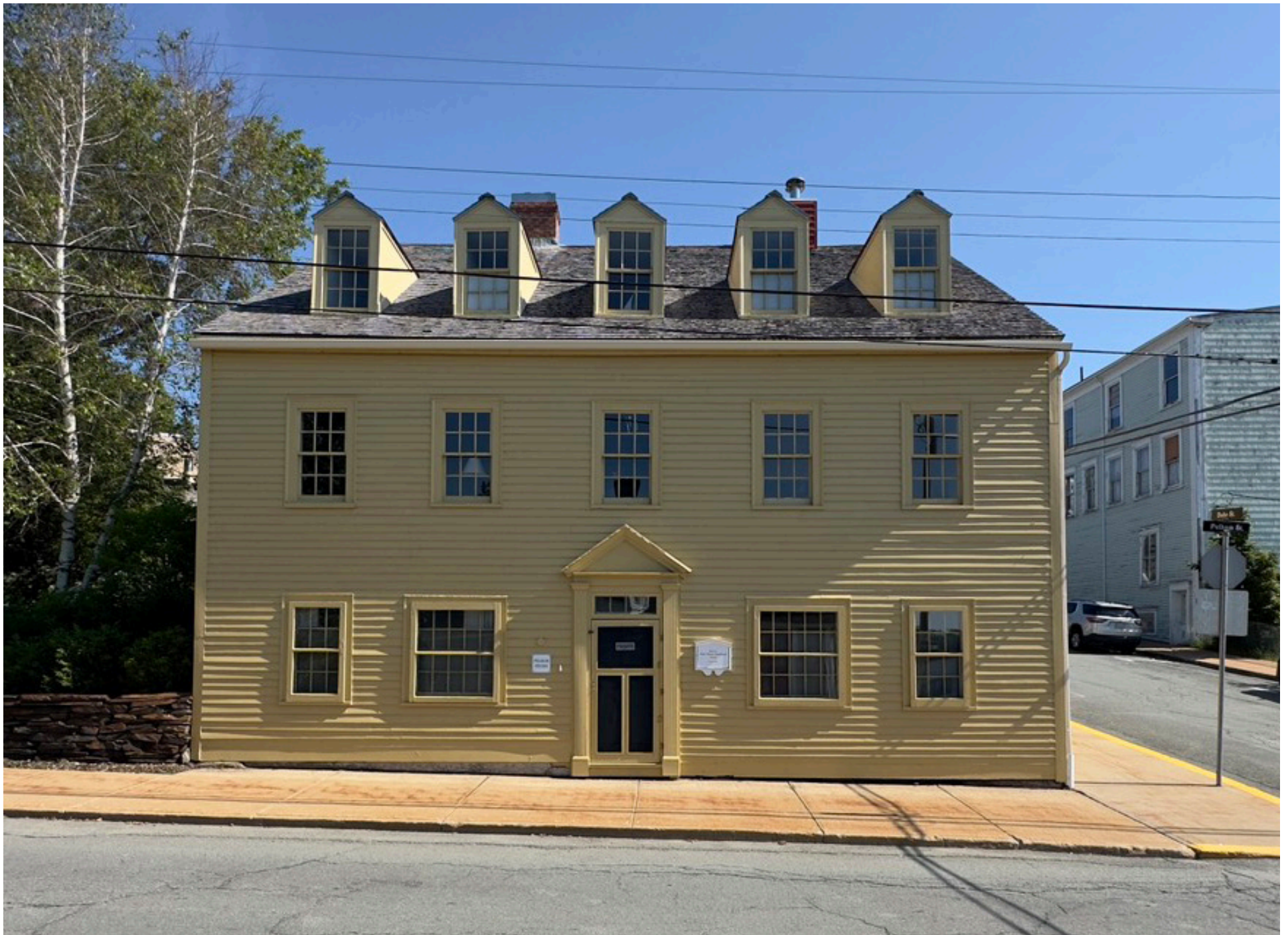
2 1/2 storey, symmetrical facade, dormers
