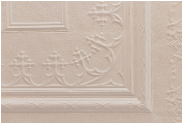
Detail views of some of the Opera House's metal ceilings.
