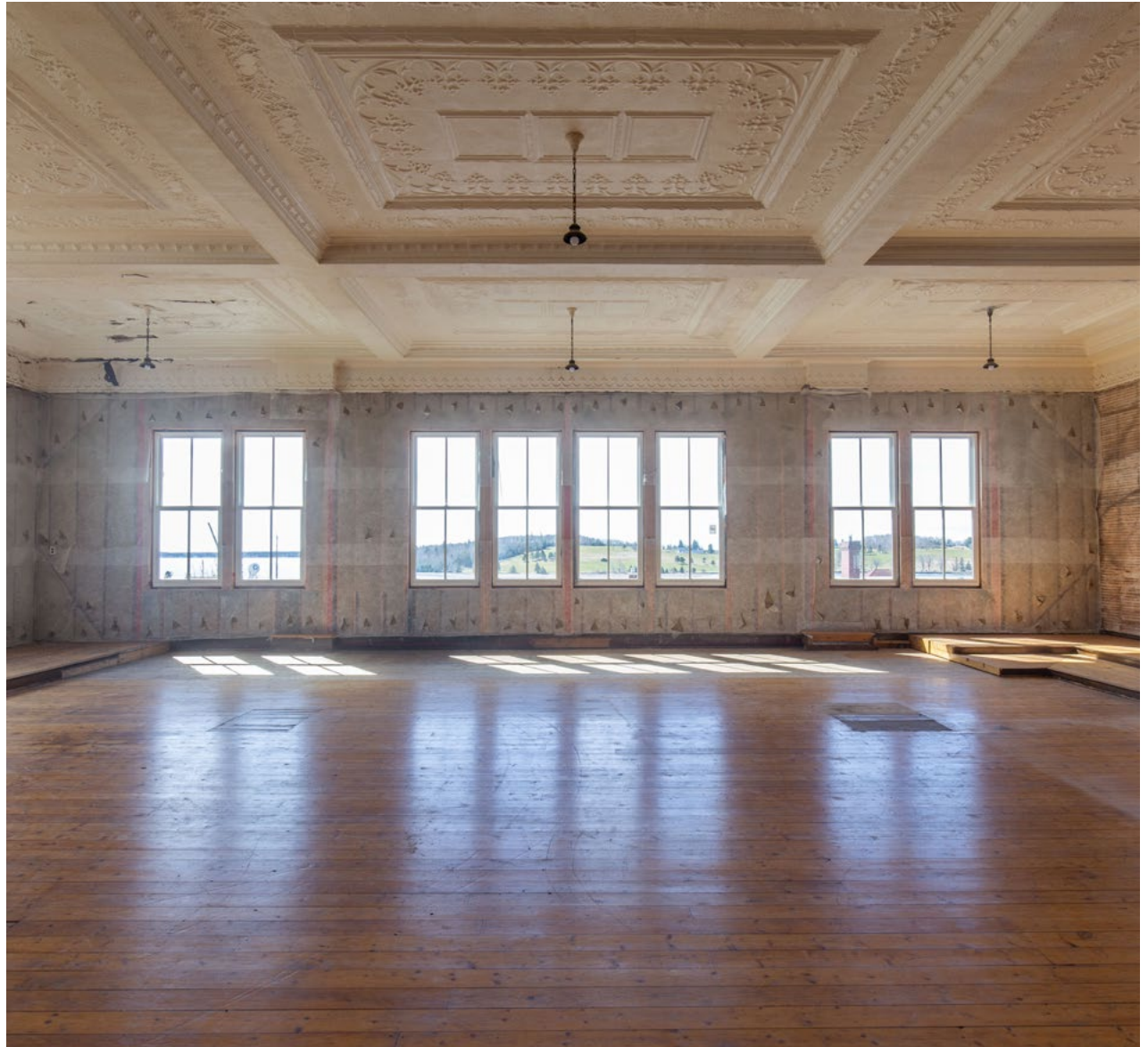
A recent image of the unfinished upper hall, proposed to become a fully accessible and safe gathering space for all.
