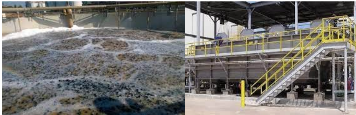
Figure 4 & 5: MBBR media and DAF unit
