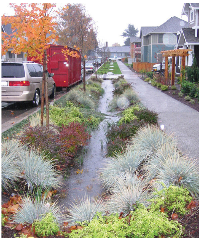
Figure 5: Bioswales collect and treat stormwater before entering the water table
