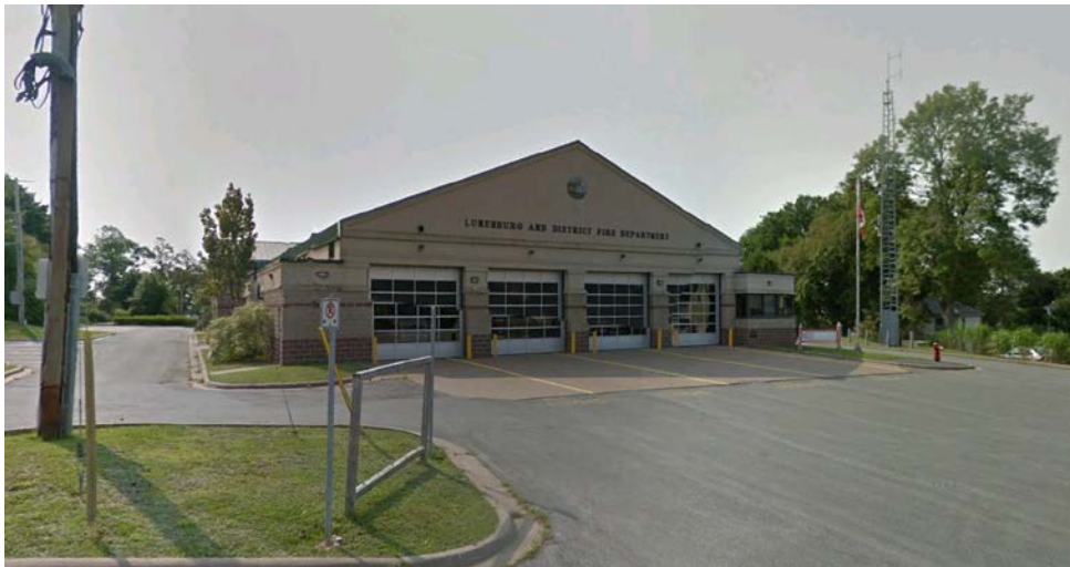
Figure 1.3: Fire station on Medway St. looking Southeast
