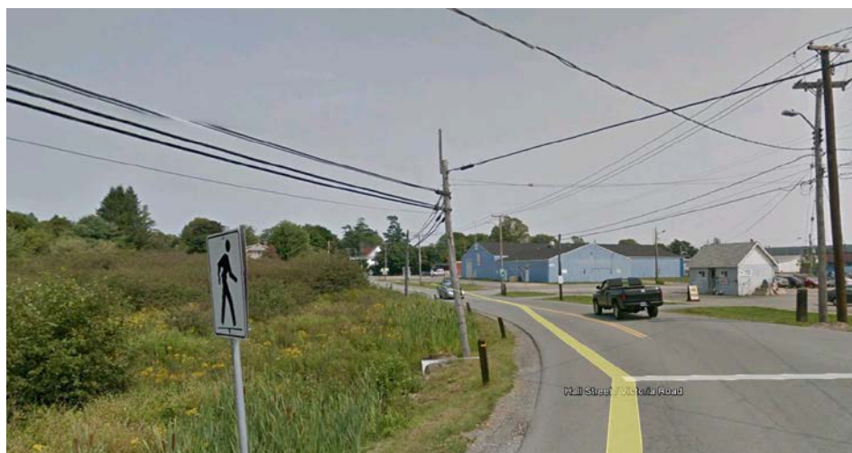
Figure 1.1: Victoria Road/Hall Street intersection looking Northeast, with the 'Blue Building' near the Community Centre in the background – Note the wetland on the left. This road regularly floods, experiencing temporary closures.
